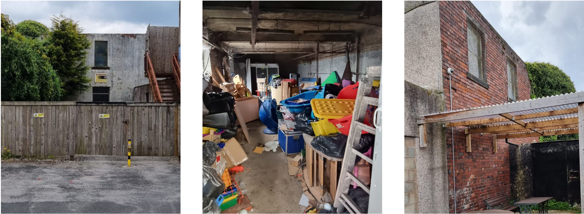
Figure 3. Existing site and building photos
