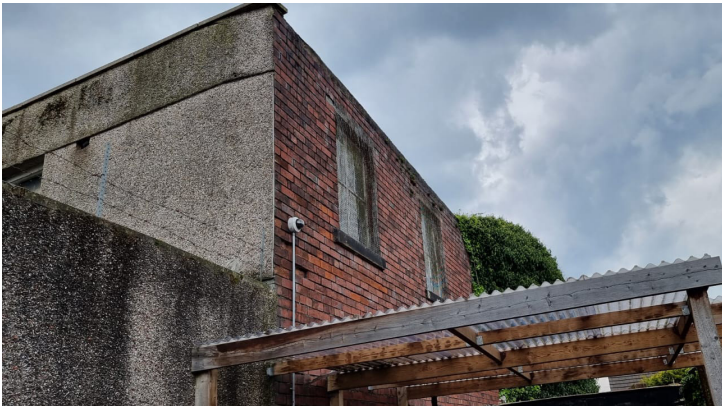
Figure 14. Existing building photos
