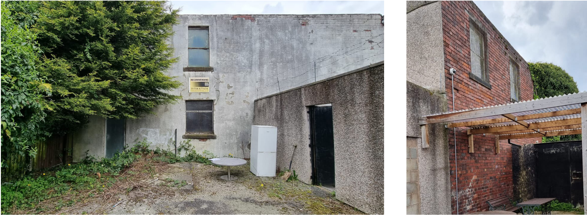
Figure 10. Existing site and building photos
