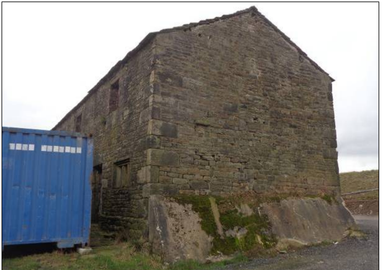
4. East gable, where projection and stack have been removed
