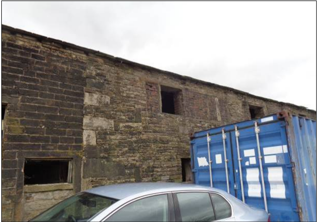
5. Long weavers' window in third and fourth bays, with quoins at end of 17 th century element
