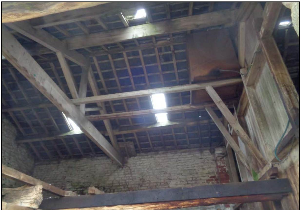
13. First bay, showing machine cut kingpost truss
