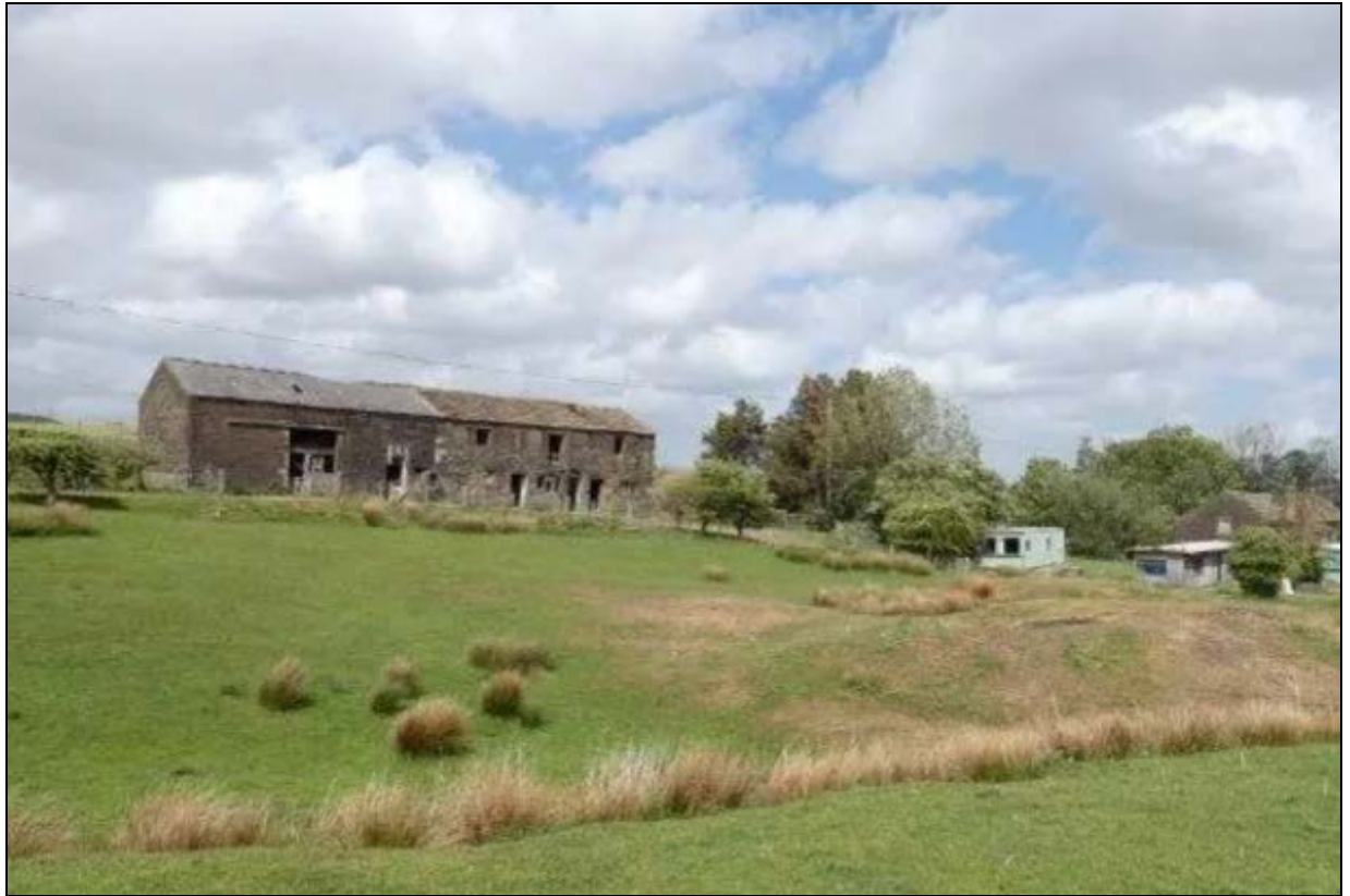
1. The outbuilding (left) forms part of the fold at Leaches Farm: view from south
