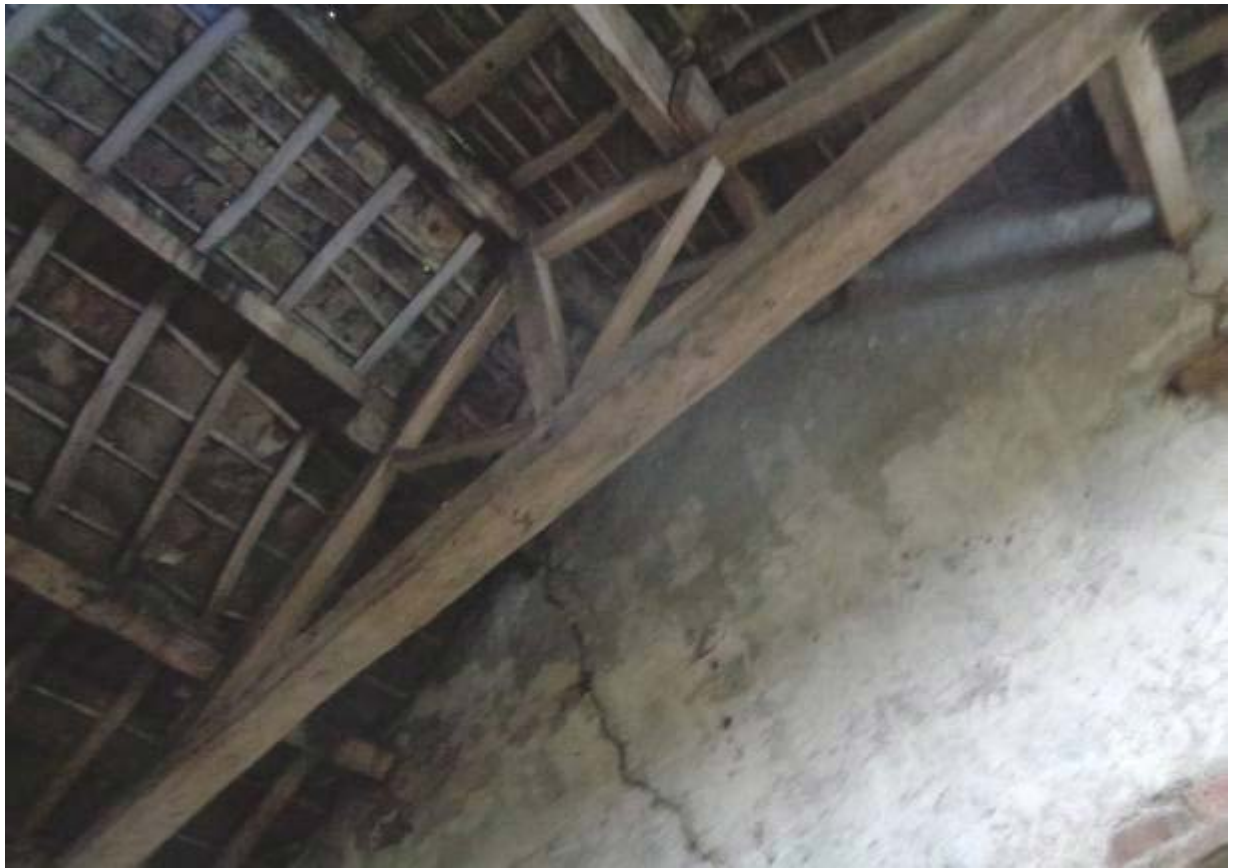
12. Truss over third bay – crosswall beyond is later
