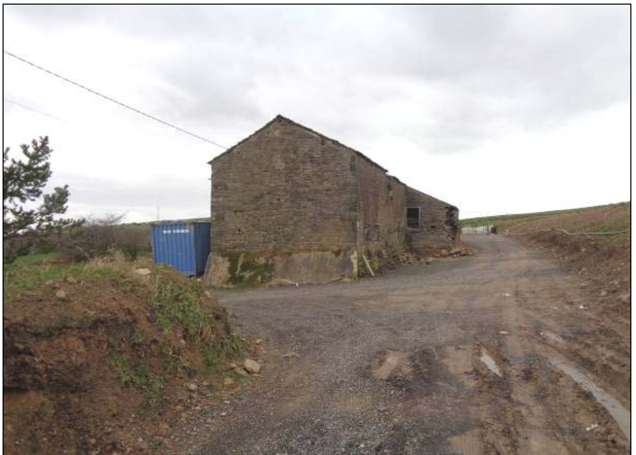
2. The outbuilding as it appears from the east
