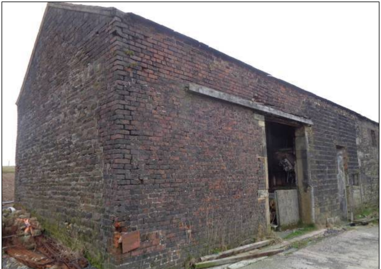
6. Fifth bay with front elevation rebuilt in early/mid 19 th century brick
