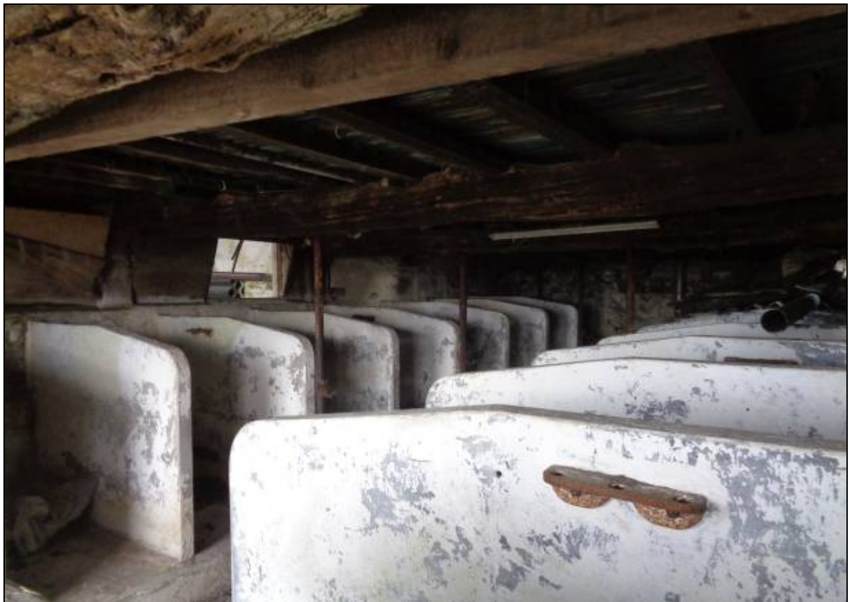
15. Interior of the second bay
