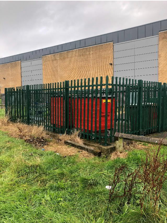
Photo 12: Fenced off bin storage
