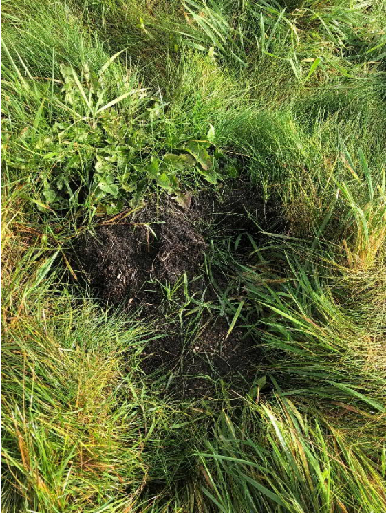
Photo 9: Evidence of infilled ground (1/2)
