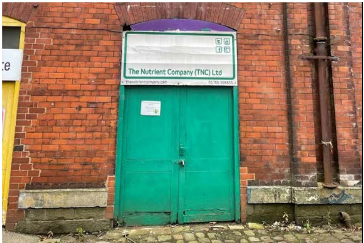
4. One of the doors in the northwest elevation
