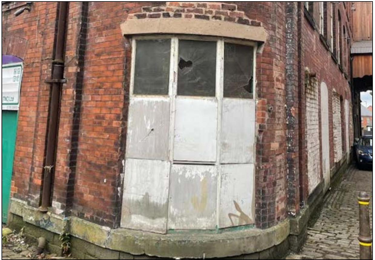
6. Window on the rounded northwest corner
