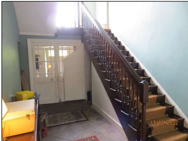
Figure 5: Photo of the existing stair with main entrance to LHS.
