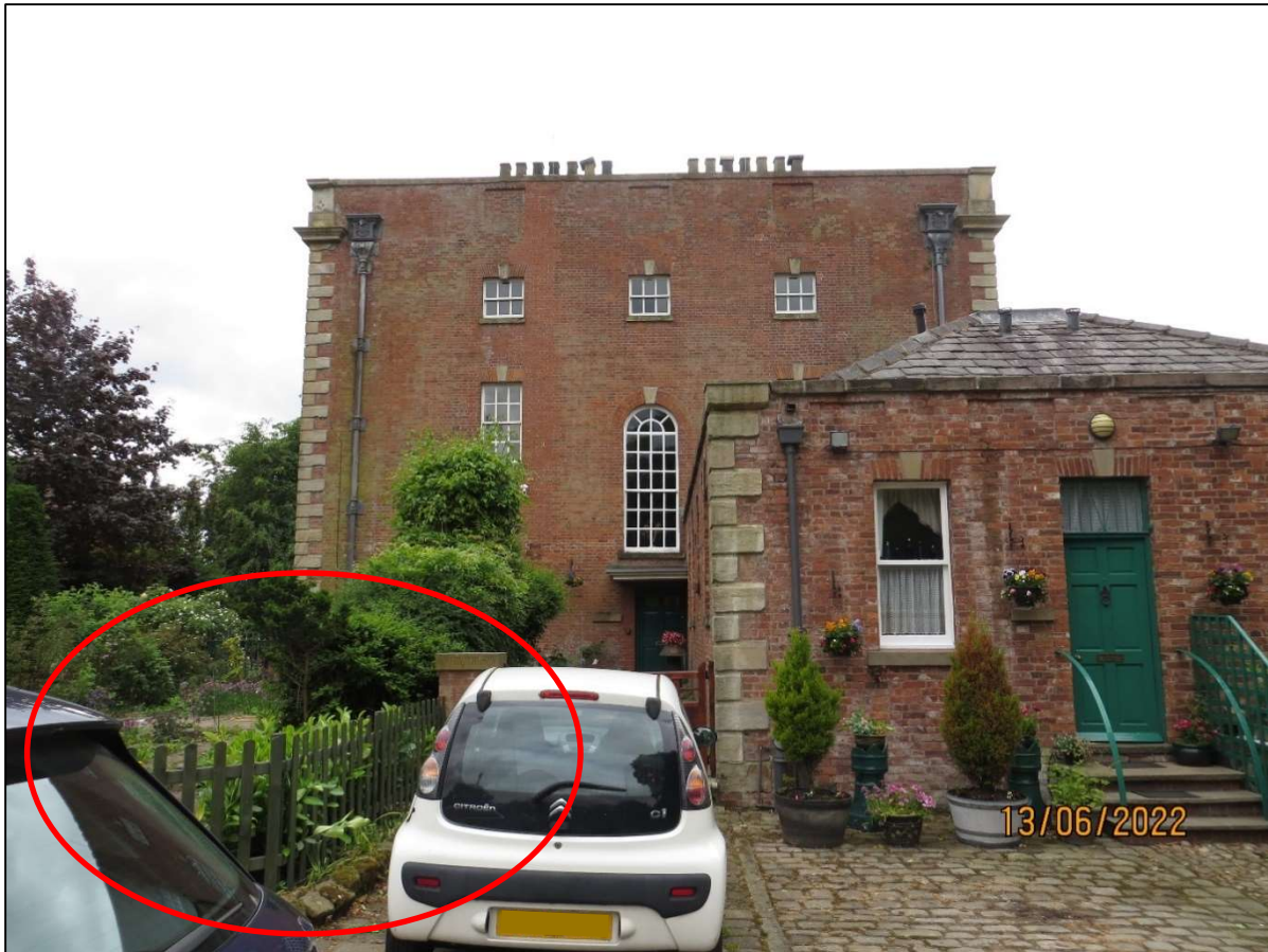
Figure 14: East elevation with main access front door for Alkrington Hall East at centre (distance). Inappropriate style and scale picket fence circled. "East Wing" separate dwelling to RHS.
