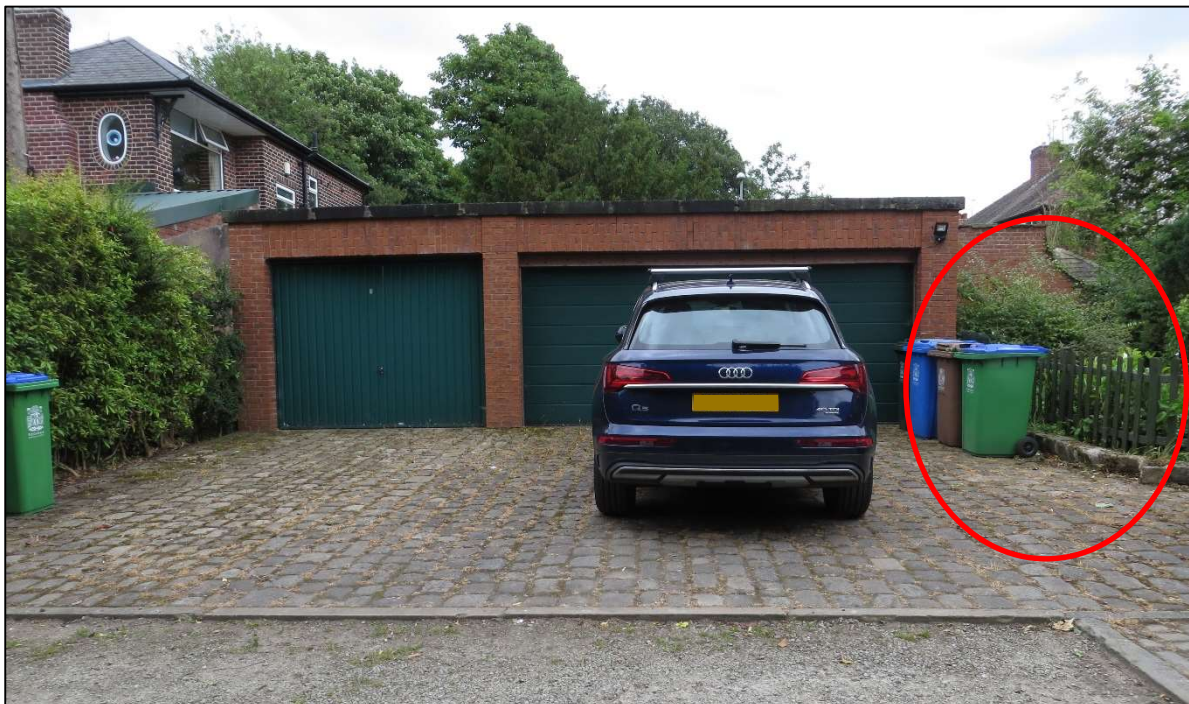
Figure 15: paved area in front of the contemporary block of flat roofed garages with lawned garden to far RHS separated by the inappropriate low picket fence (circled).
