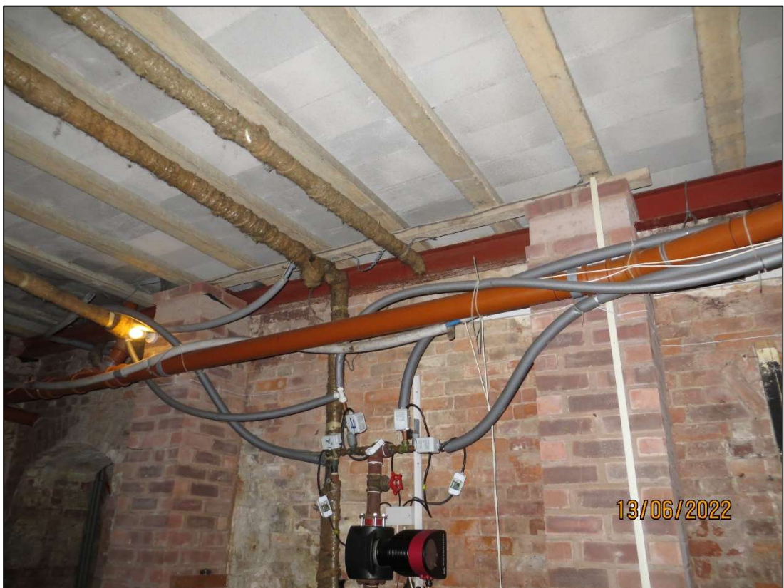
Figure 9: The existing basement space where the proposed stair will be. The new opening will be formed in the non-original concrete floor of the hall above.
