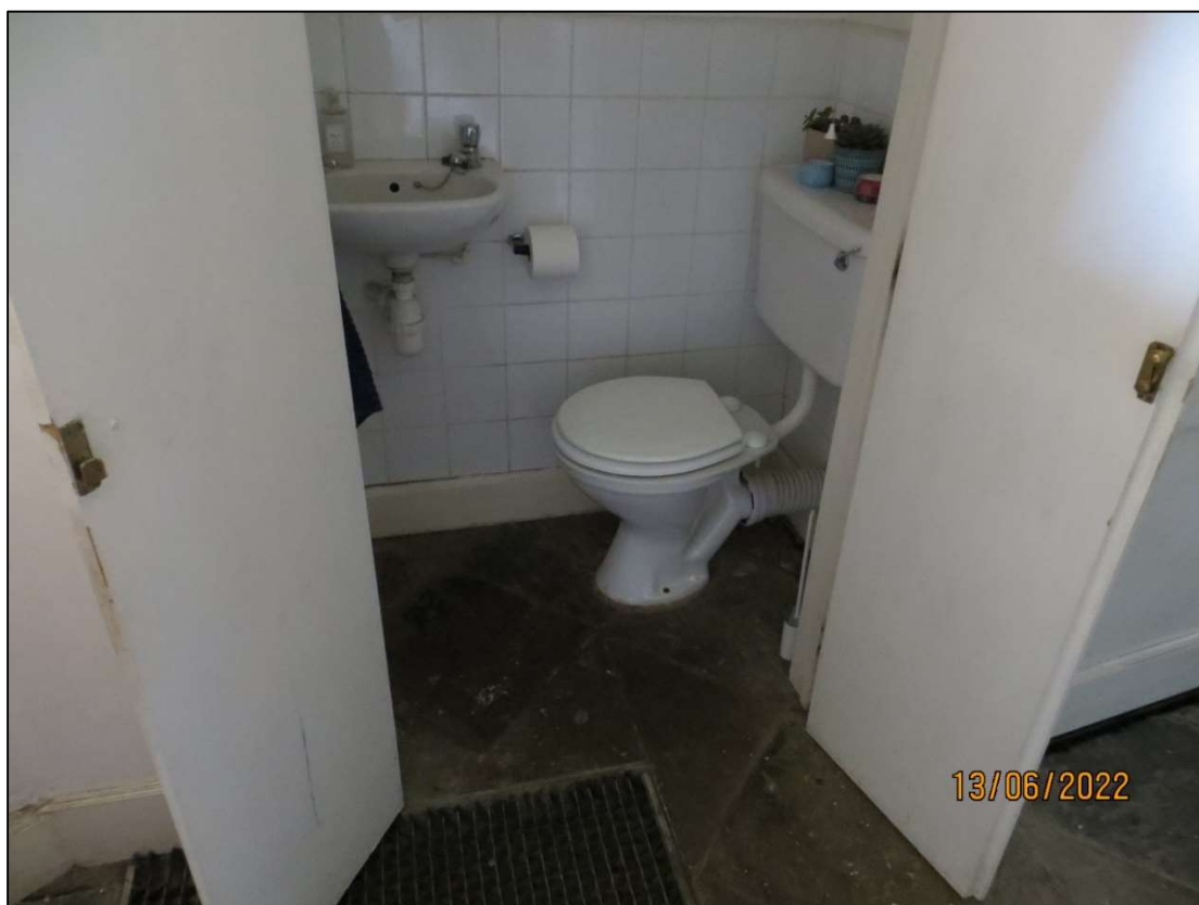
Figure 7: Photo of the WC under the stairs within the main entrance lobby. The head of the new stair will be within this space behind a door.
