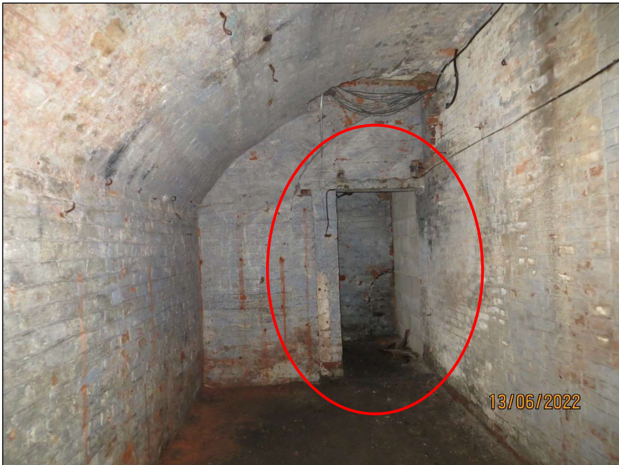
Figure 12: The connecting open doorway through to the adjacent "East Wing" dwelling basement space. The proposal is to put a lockable door in this existing opening.
