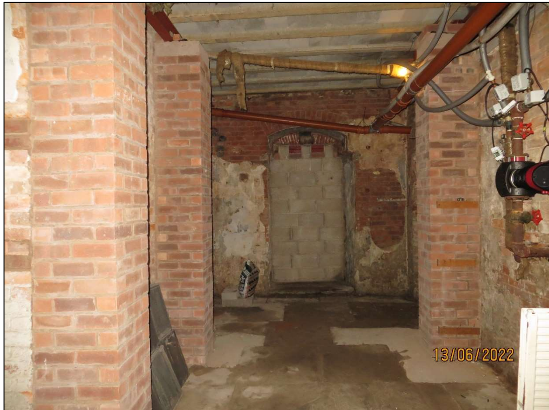
Figure 8: The existing basement space where the proposed stair will be with the foot of the new stair in the foreground. Note the non-original concrete ceiling (which is the floor of the hall above) and modern supporting brick piers and steel beams.
