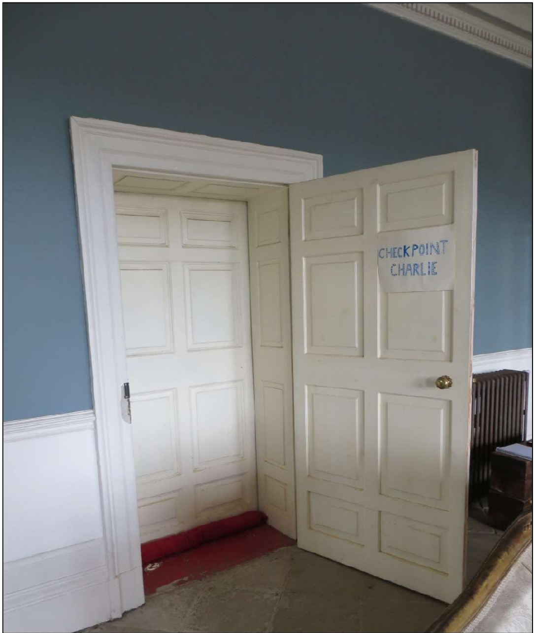
Figure 11: The connecting door through to the adjacent dwelling opened revealing the second door through to the adjacent property of Alkrington Hall West and the small space between with the panelling detail.
