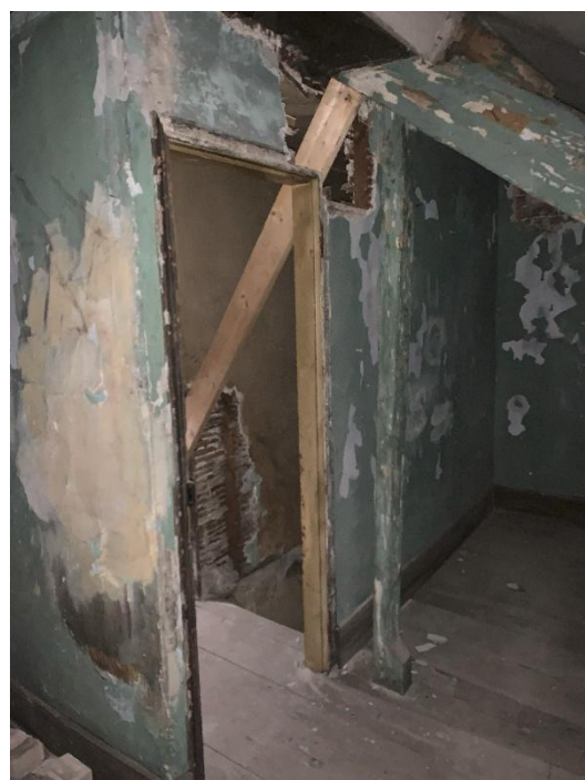
Figure 2.7: Vestibule in the roofspace.
