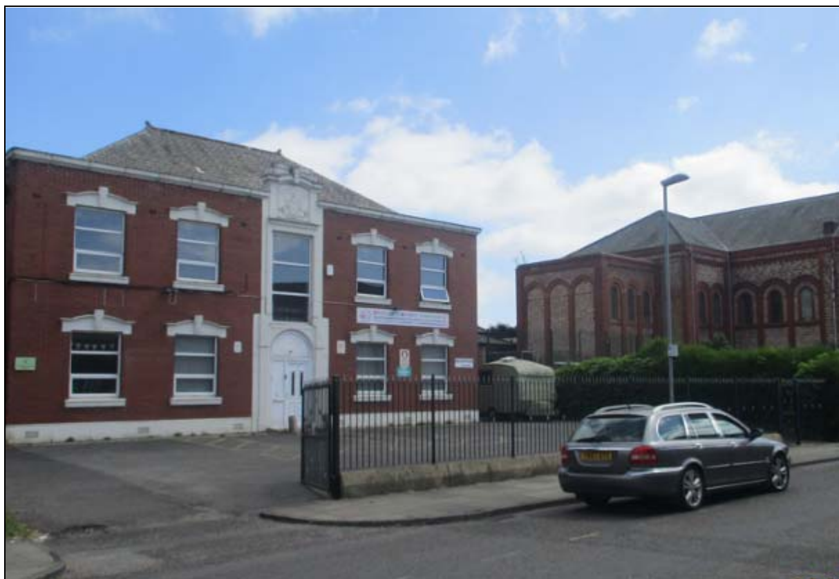
The front elevation is a distinctive feature of the Taylor Street streetscene
