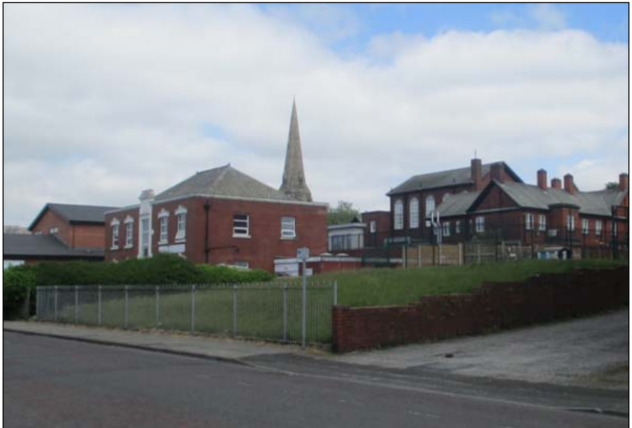
The building within the Taylor Street streetscene
