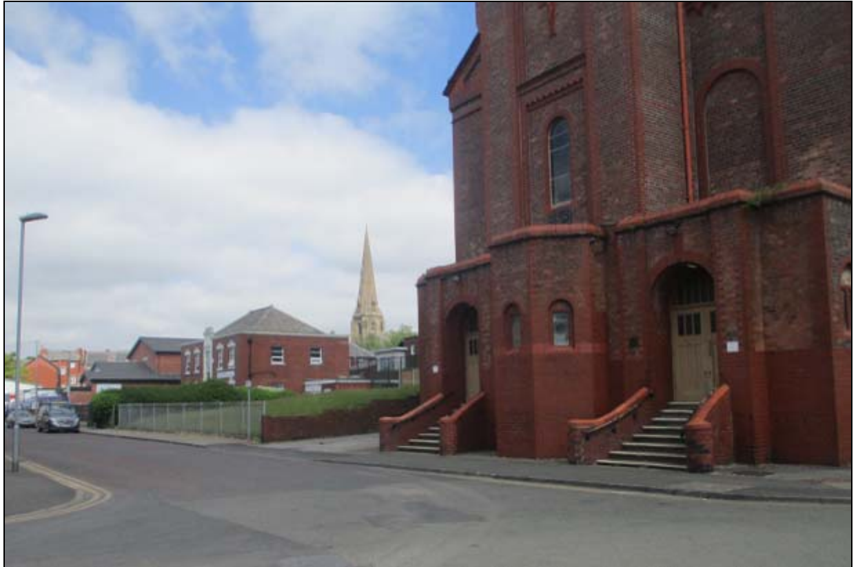
The church is the predominant building amid its immediate surroundings
