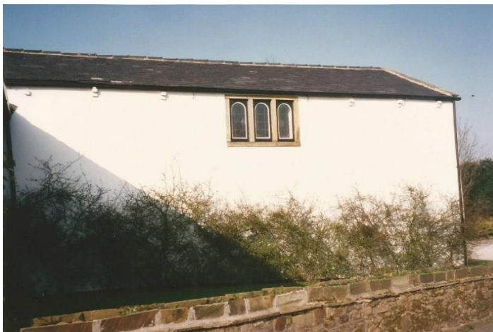
C17 barn "The Workshop" facing East photo taken in 1981
