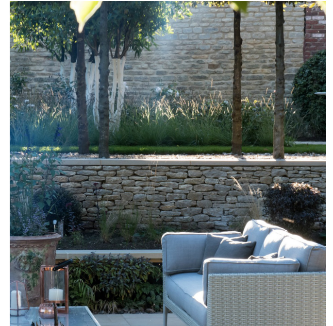
4. Yorkstone Retaining Wall
