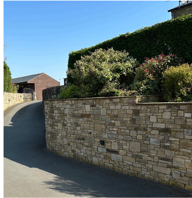
2. Existing Wall Retained
