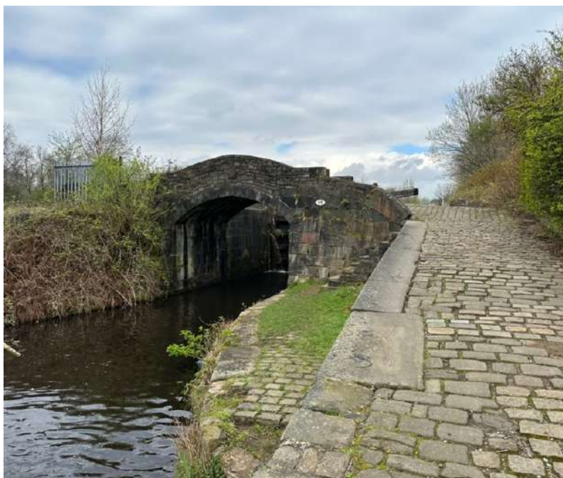
Figure 4.1: Rochdale Canal Lock No 52 and Towpath Bridge (April 2024)
