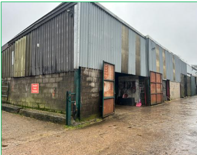
The south and west elevation of the stable block
