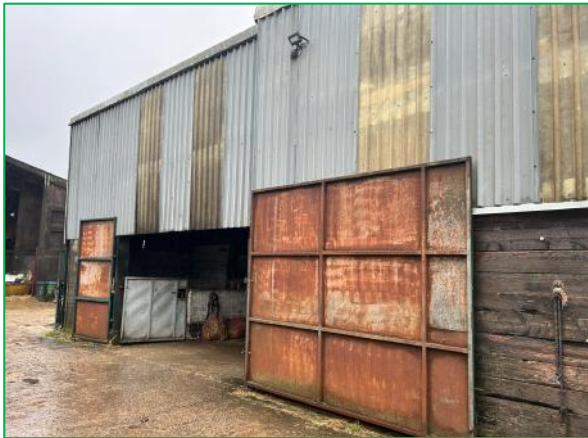
The south elevation of the western end of the stable block
