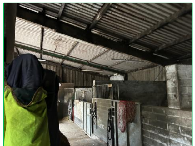
The internal space in the western half
