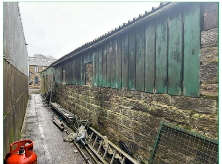
The north elevation of the stable block
