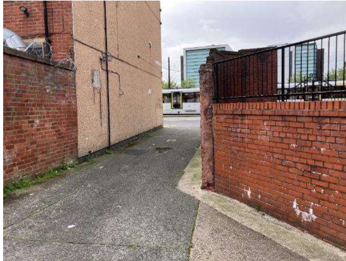
Figure 25 – View on Fire Station Yard to the North of the Existing Building
