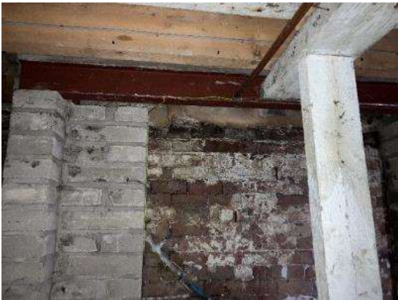
Figure 12 – Steel Support Under Main Entrance Above
