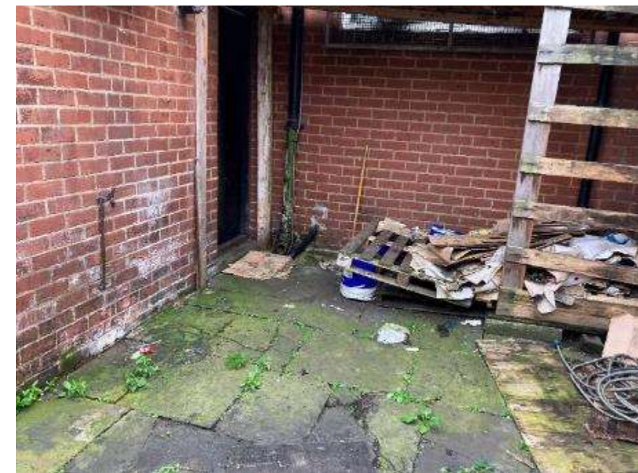
Figure 21 – View on Rear Access Door Via Yard Area
