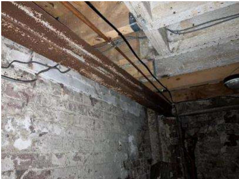
Figure 11 – Steel Beam Supporting Joist Ends
