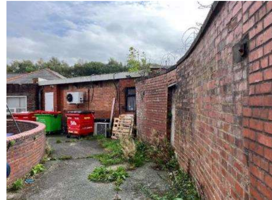
Figure 23 – View on Unnamed Access Road to Rear
