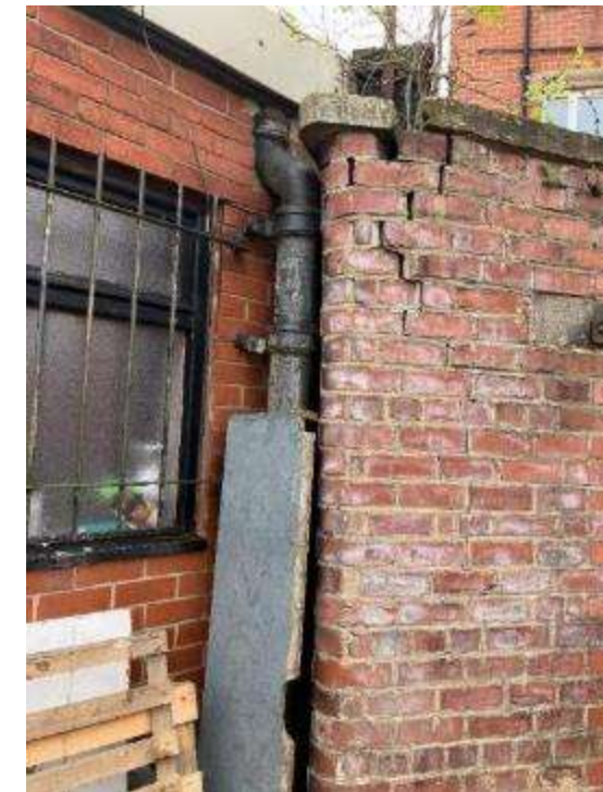
Figure 24 – View on Junction with Adjacent Singlet Storey Building
