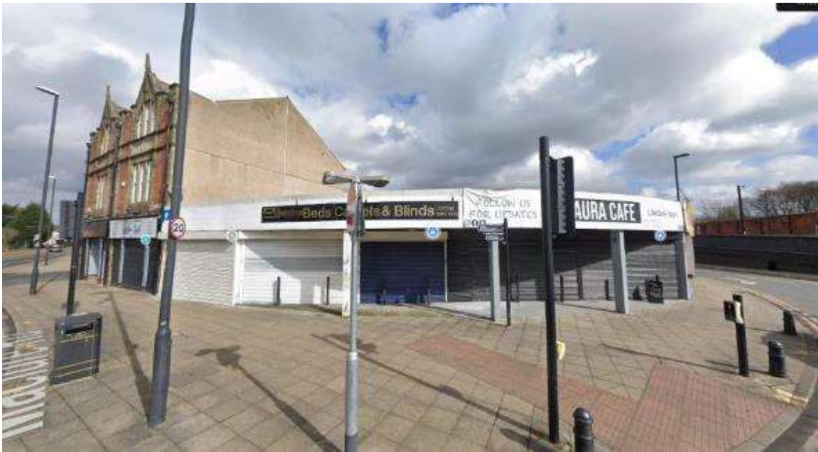
Figure 2 – View on Existing Buildings (Looking North)
