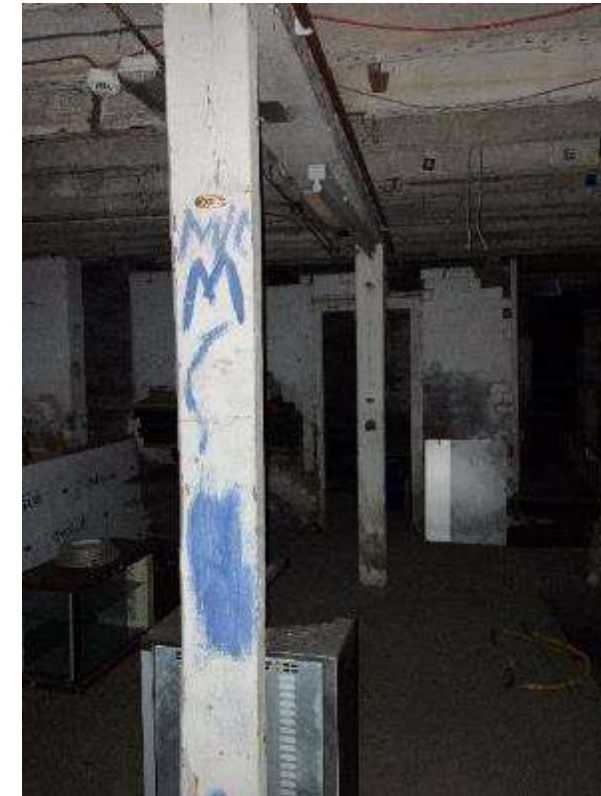
Figure 9 – Possible Historic Floor Strengthening Members
