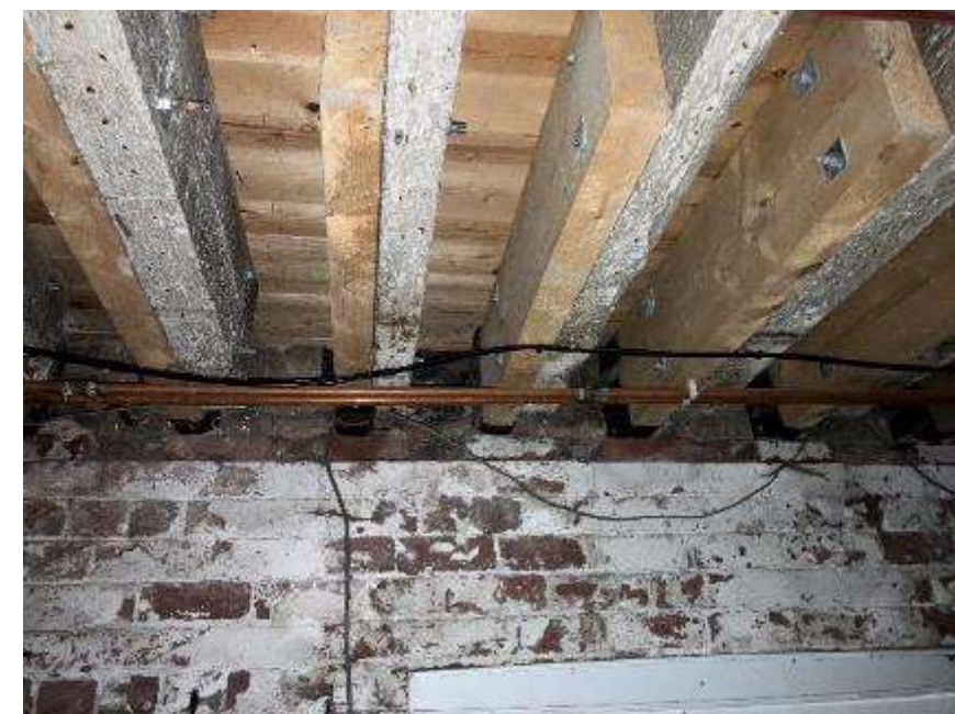
Figure 10 – Historic Timber Repairs to South Gable Wall
