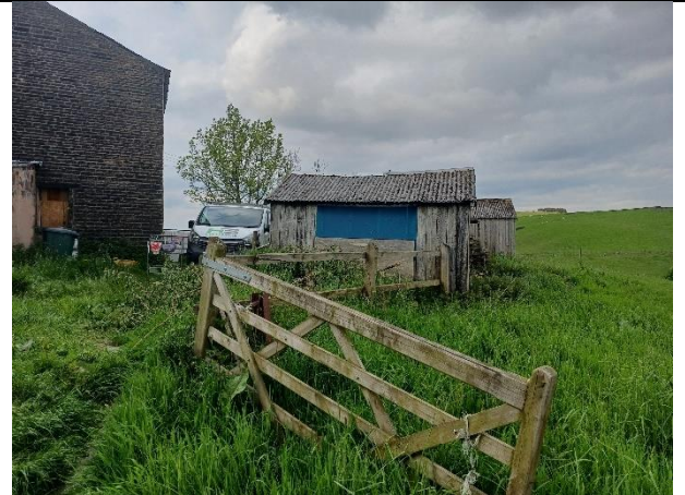
Photograph 4: The majority of the outbuildings had what appeared to be corrugated asbestos cement roofs.
