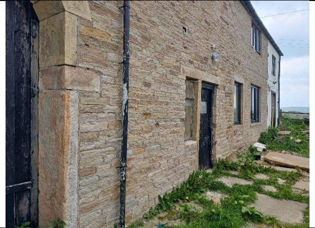
Photograph 2: Sandstone Farmhouse building with flagged small courtyard area.
