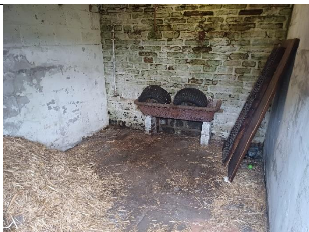
Photograph 11: Packed earth floor beneath the hay within the outbuilding. Mossy stonework but no sign of efflorescence or chemical attack.
