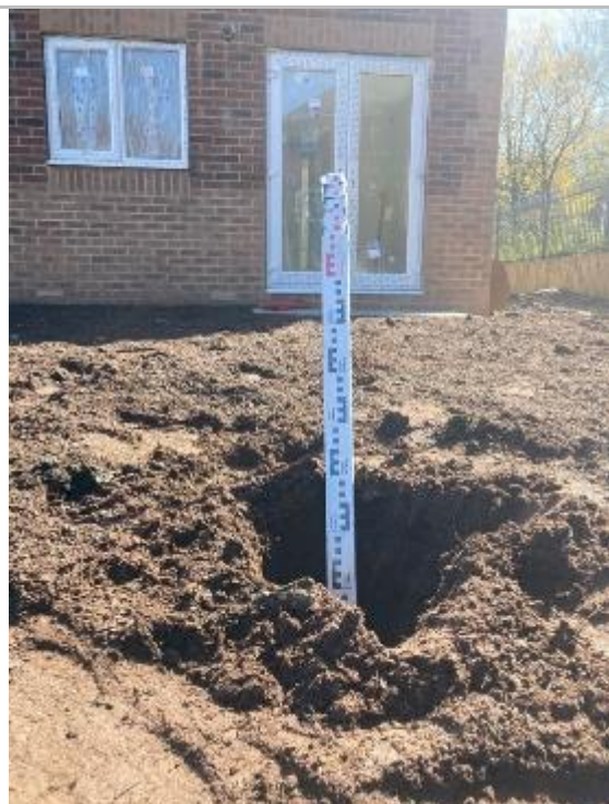
Depth of Cover System at Ground Level
