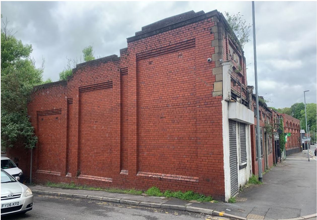
Photograph No 2: View of Southern Elevation Pre-Demolition
