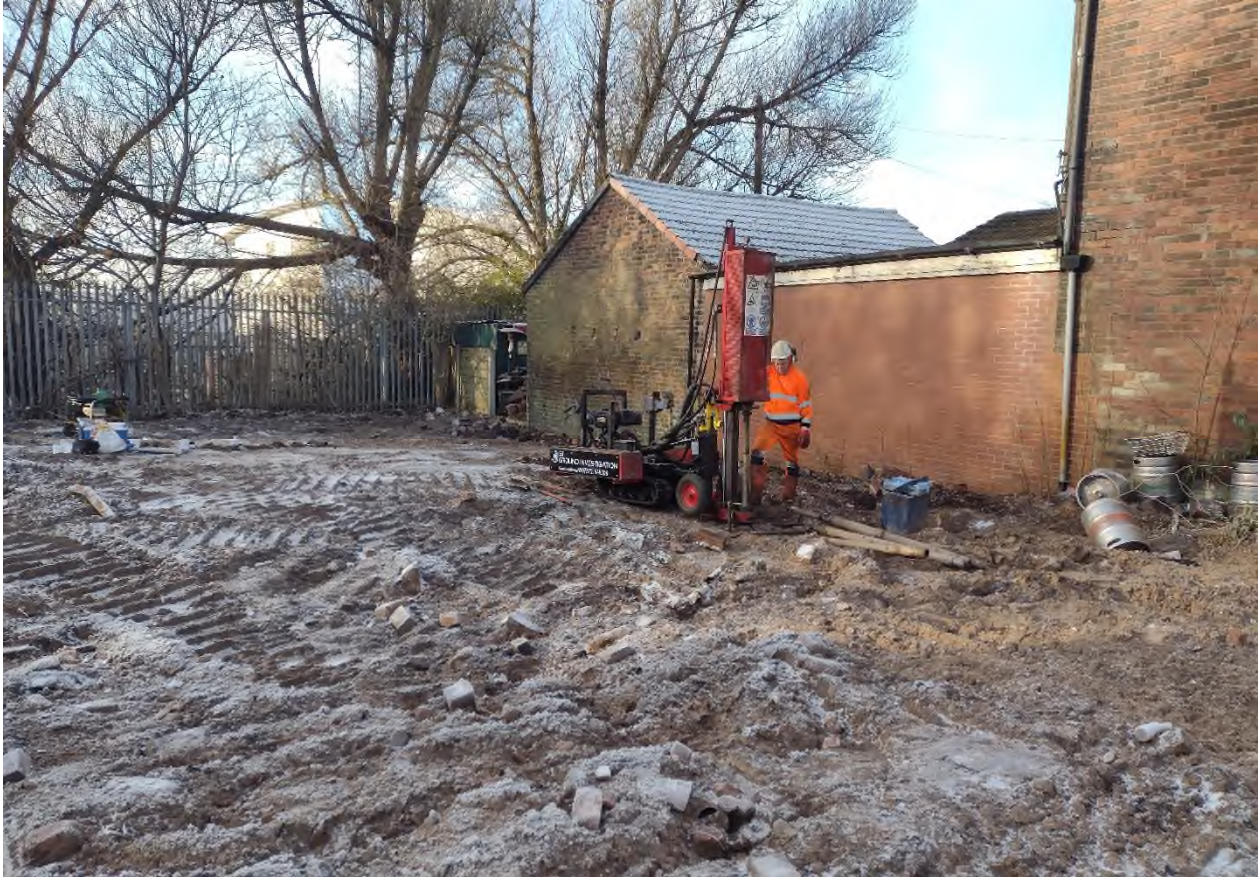
Photograph No 7: Drilling Borehole No 2
