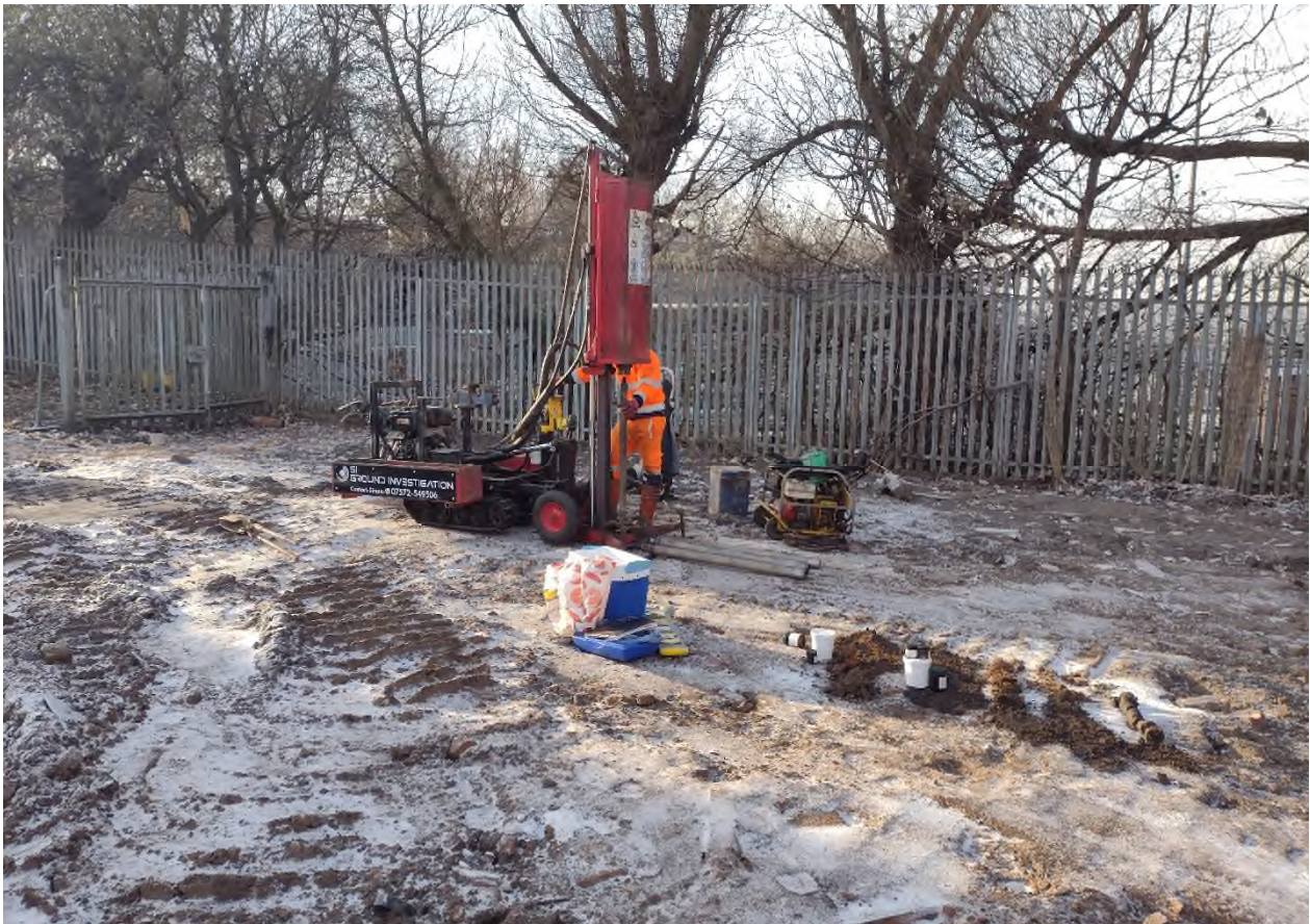
Photograph No 8: Drilling Borehole No 3/3A
