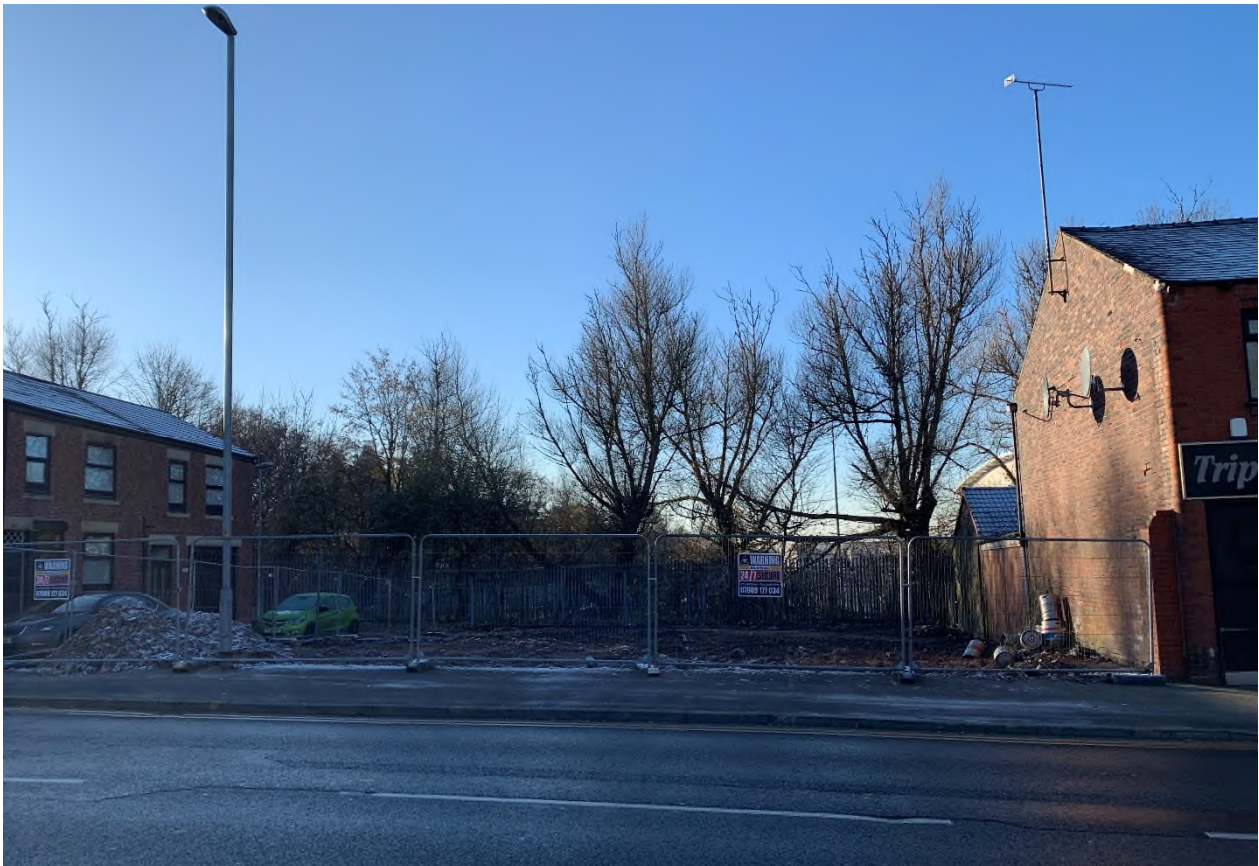
Photograph No 4: View from Townley Street Post Demolition
