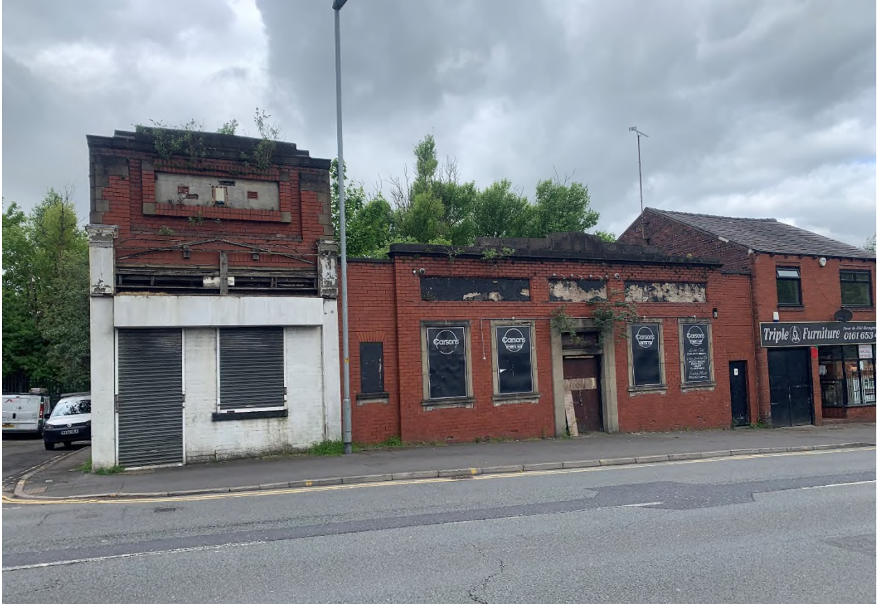
Photograph No 1: View from Townley Street Pre-Demolition
