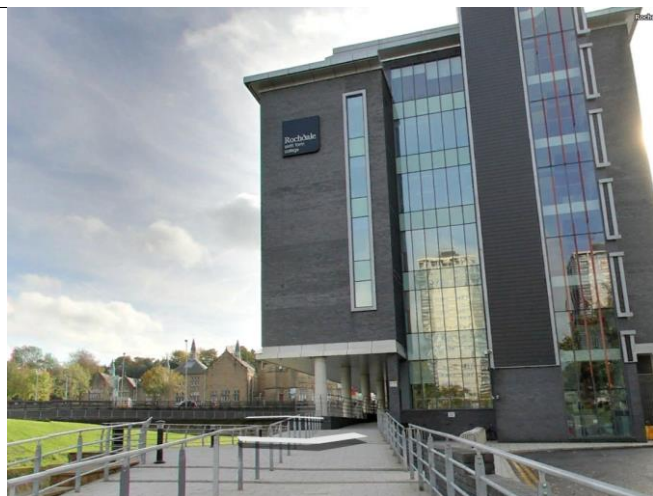
Photo 13: Northern elevation of the existing building; 'negligible' suitability for use by roosting bats
