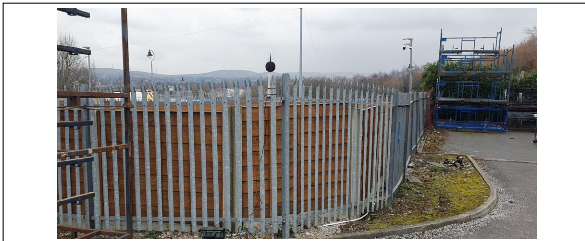
Figure 3: Site Location Measurement Pictures
