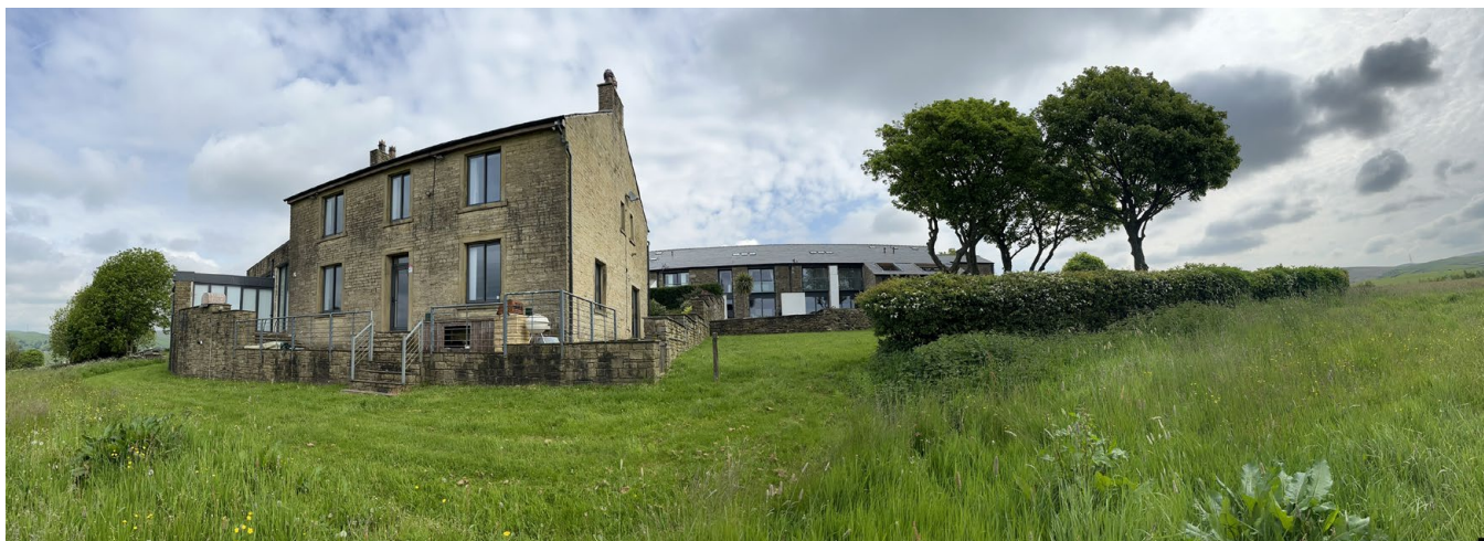
SITE CONTEXT 1 - THE SOUTHERN ELEVATION OF THE FARMHOUSE WITH THE NEIGHBOURING CONVERTED BARN IN BACKGROUND
