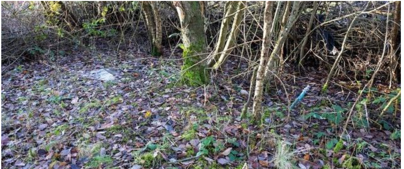
Figs. 9 & 10. Compound Water Supply (Blue Alkathene pipe) & Drainage Pit Cover .
