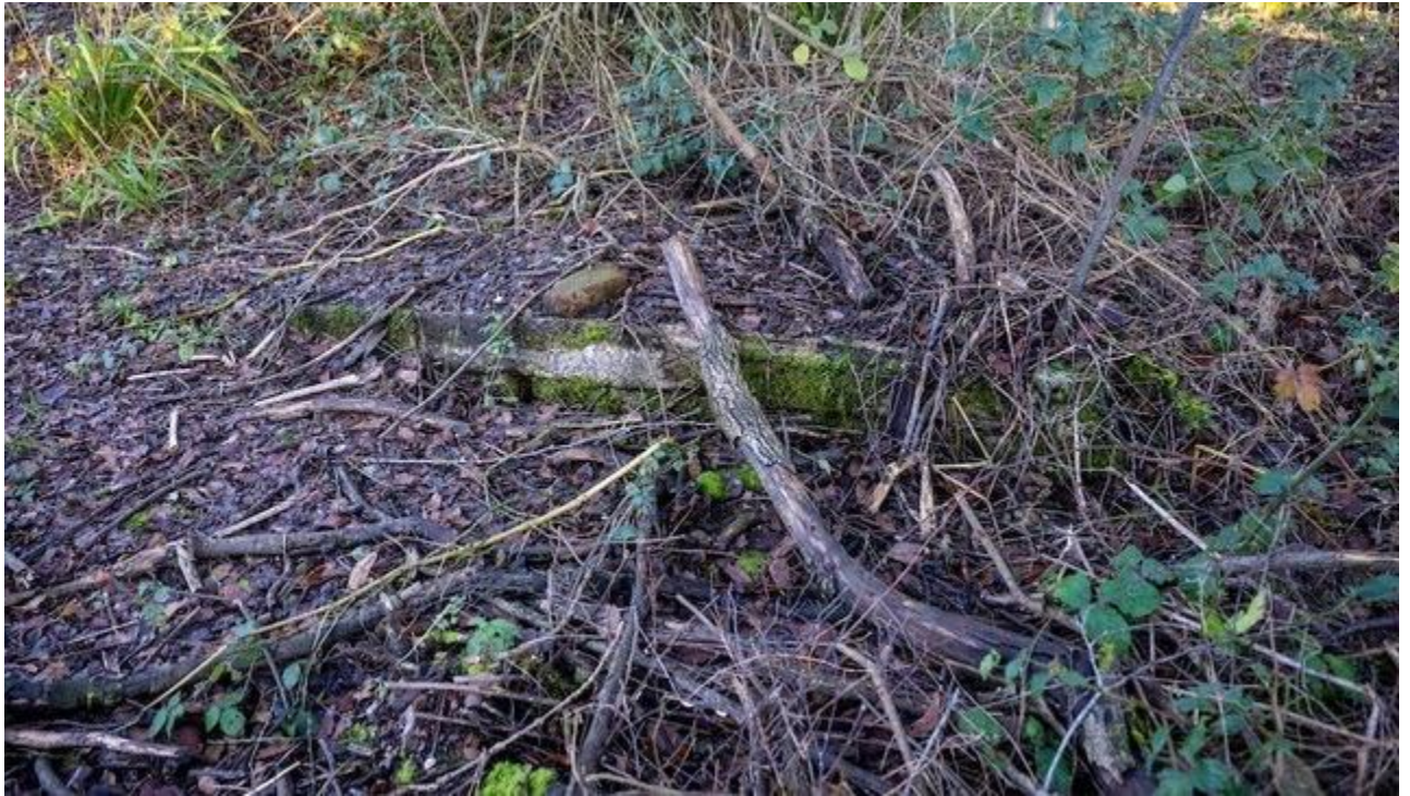
Fig. 5. Concrete Base Slab of Previous Centre.
