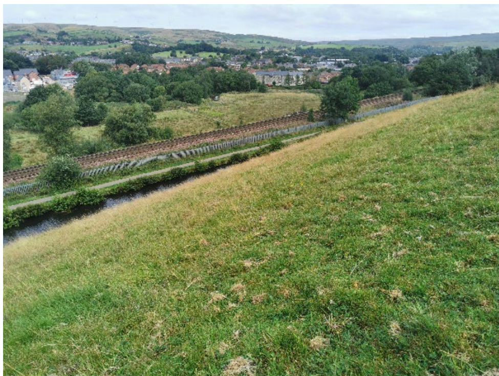
View of slope to canal
