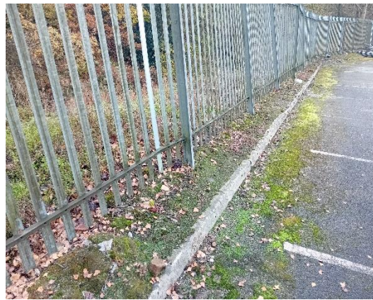
Photo 2: Strip adjacent kerb at base of palisade fence beyond hard standing area
