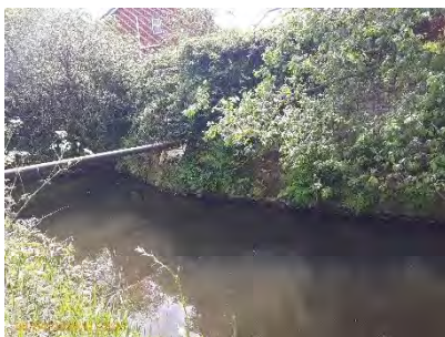
Figure 6: Steep densely vegetated banks - Section D
