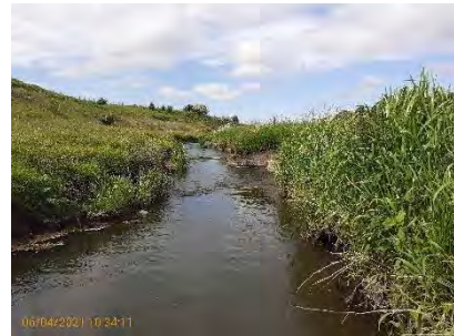
Figure 3: Section A - Densely vegetated banks
