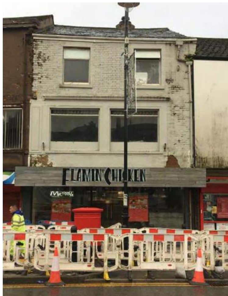
Above: Shopfront prior to renovations and HAZ development.
