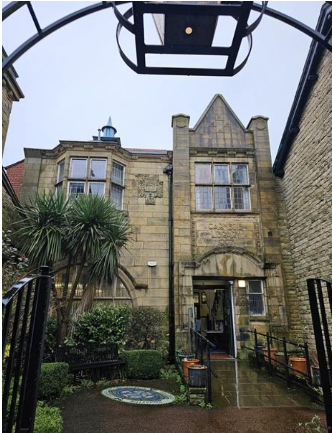
1. Milnrow Library – front elevation (Section 1)
