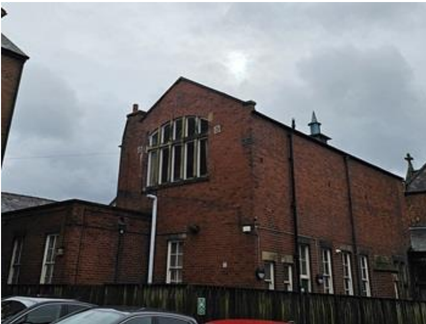
2. Section 2 (to right) with flat-roofed Section 3 (to left) – northwest and northeast elevations
