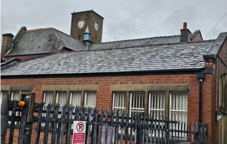
3. Section 2 (foreground) and Section 1 behind – southeast elevations
