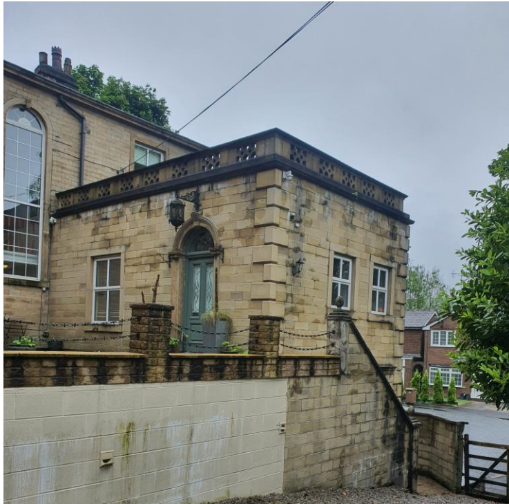
Figure 5: Existing Extension on West Elevation of Bentgate House
