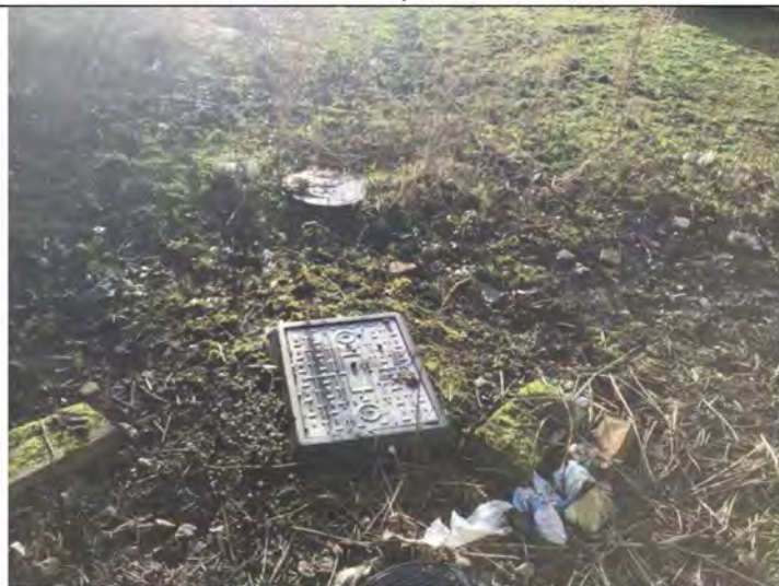
Photograph 5 (P5) Manhole covers associated with soakaways in the west.
