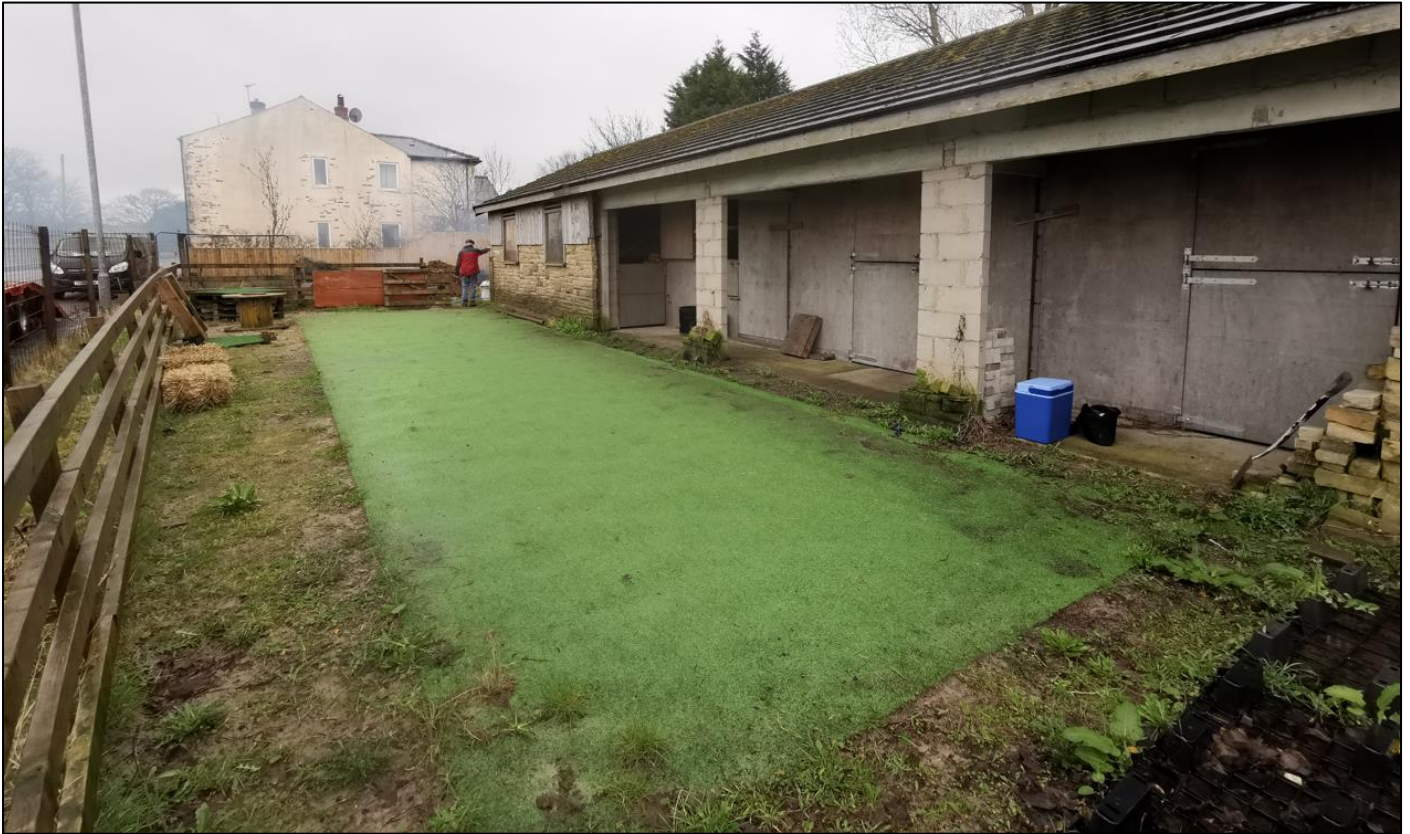
General Site photo from NW Site corner to E.
