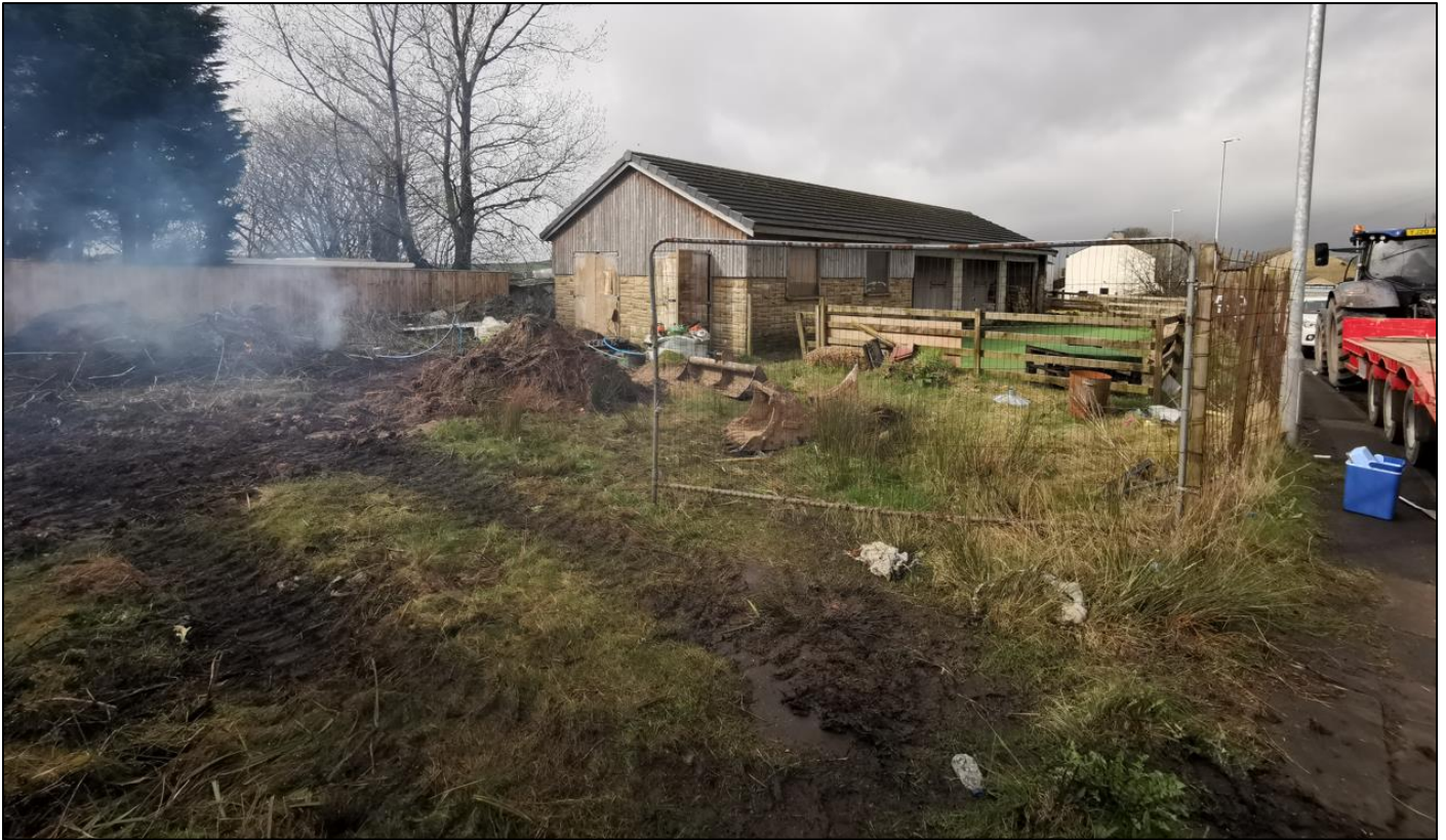
General Site photo from NE Site corner.
