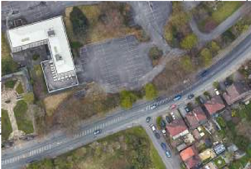
NORTH SOUTH AERIAL VIEW
