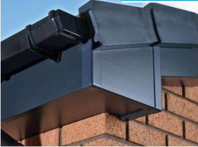
Black uPVC fascias, soffits and barge boards with black gutters and downpipes.
