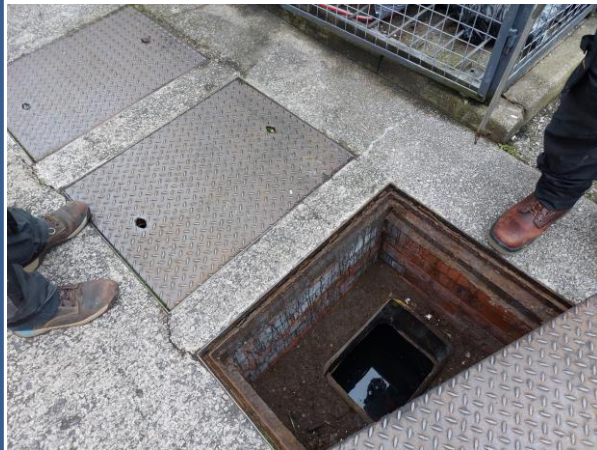
Image 4: Three stage interceptor, near car wash building. First stage shown.
