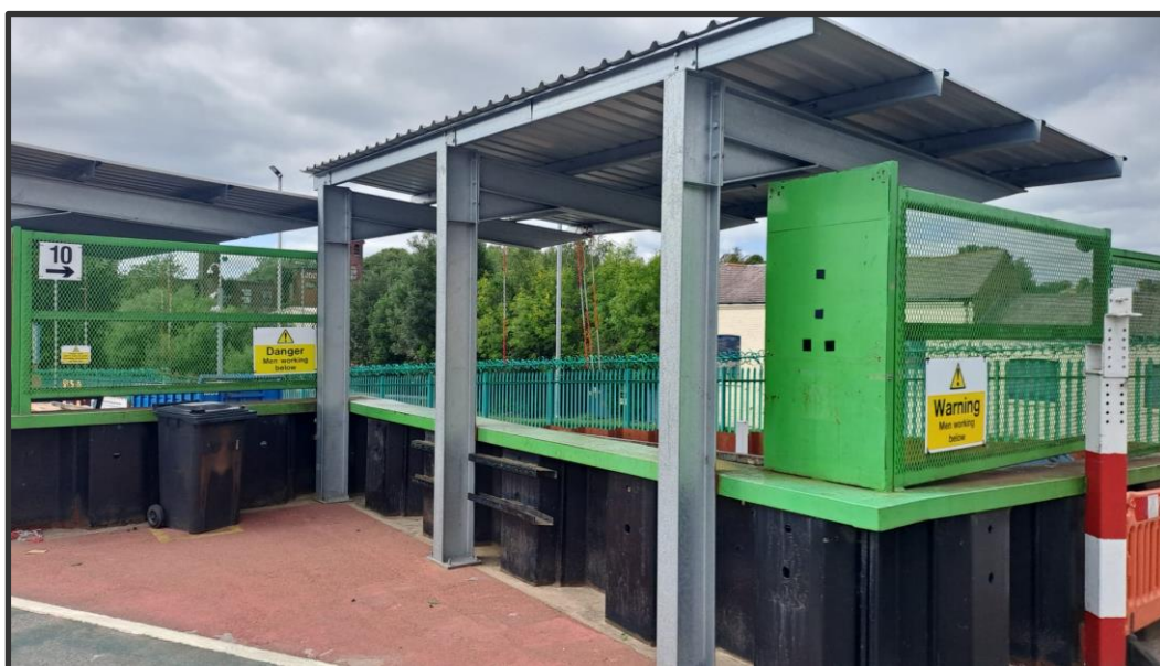
Figure 1 – Photographs of the canopies
