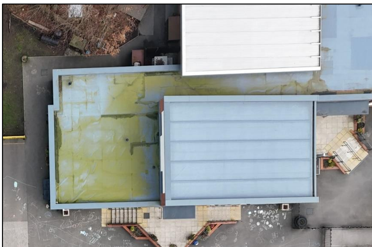
Photograph 6 showing the part of the building to be extended
