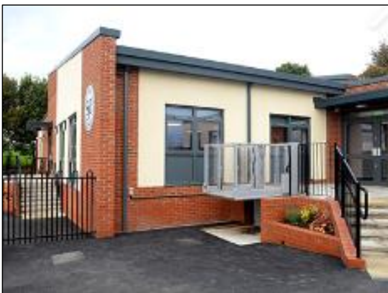
Photograph 3 showing the newer portion of the building.
