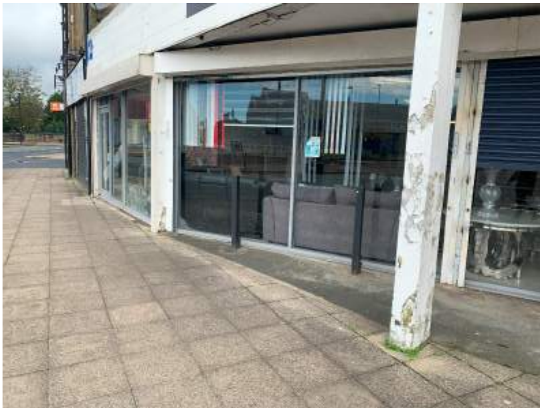
Plate 4 – Single storey building on site hosting vacant units, looking north.
