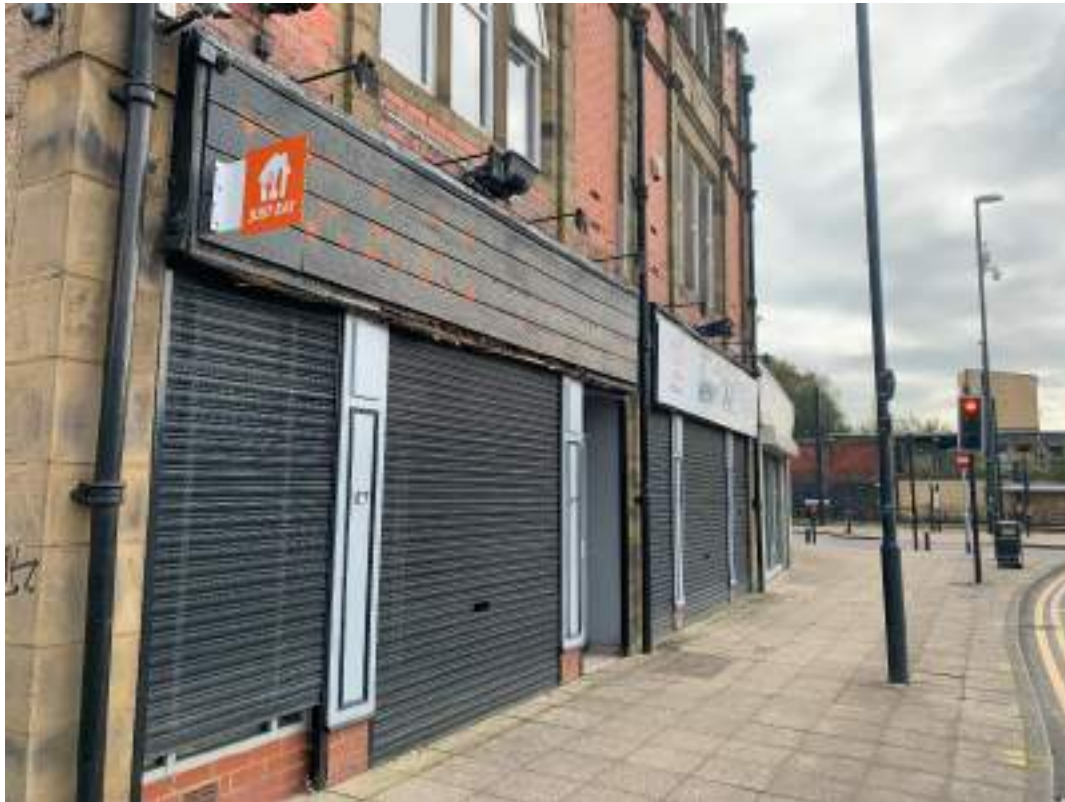
Plate 3 – 3-storey building present on site, looking south.
