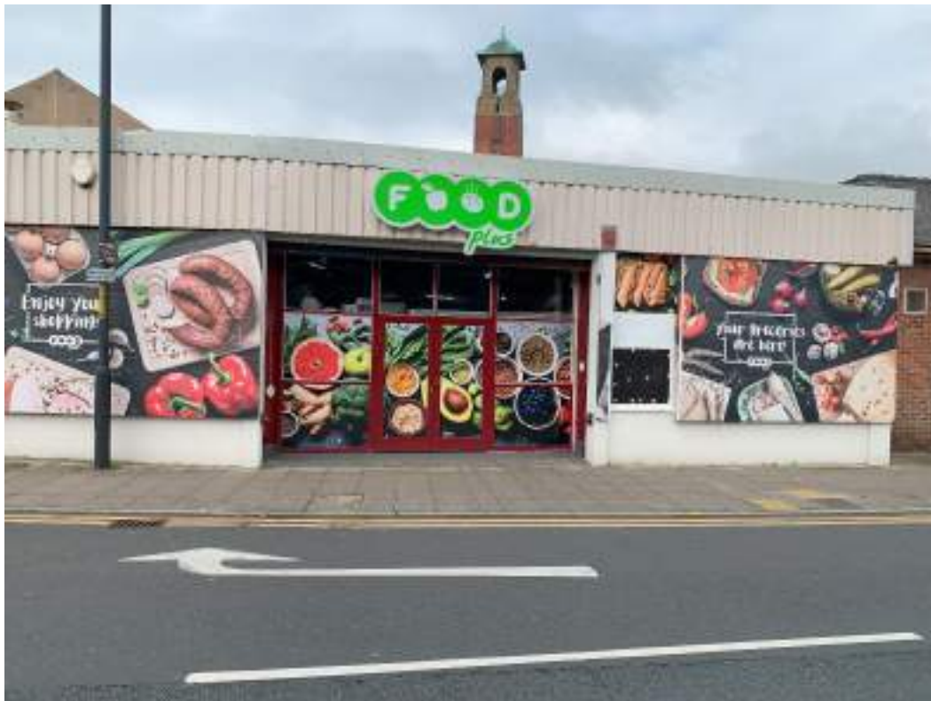
Plate 5 – Existing retail unit in the east of site, looking north.
