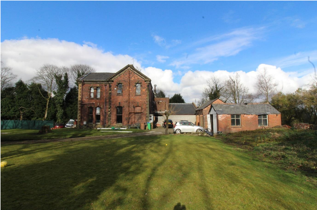
Plate 9 – Site from side
