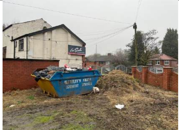
P2: A metal skip filled with household waste and a soil stockpile in the eastern corner of the site.
