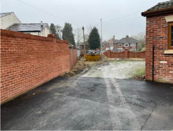
P1: A view looking east across the site
