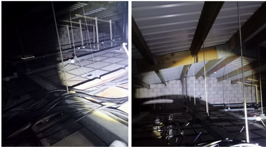
Figure 5 The loft space of the property at Bowlee Park Driving Range, Heywood Old Road, Middleton M24 4TH, Near Rochdale
