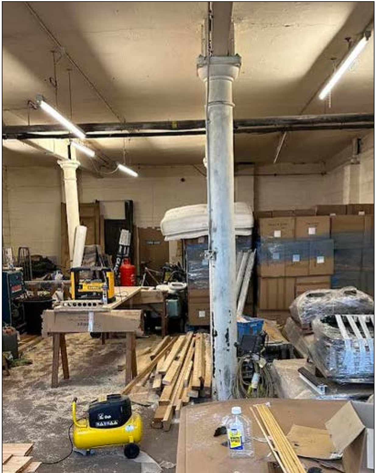
6. View through unit 30 showing cast iron columns principal space of the unit, looking northwest
