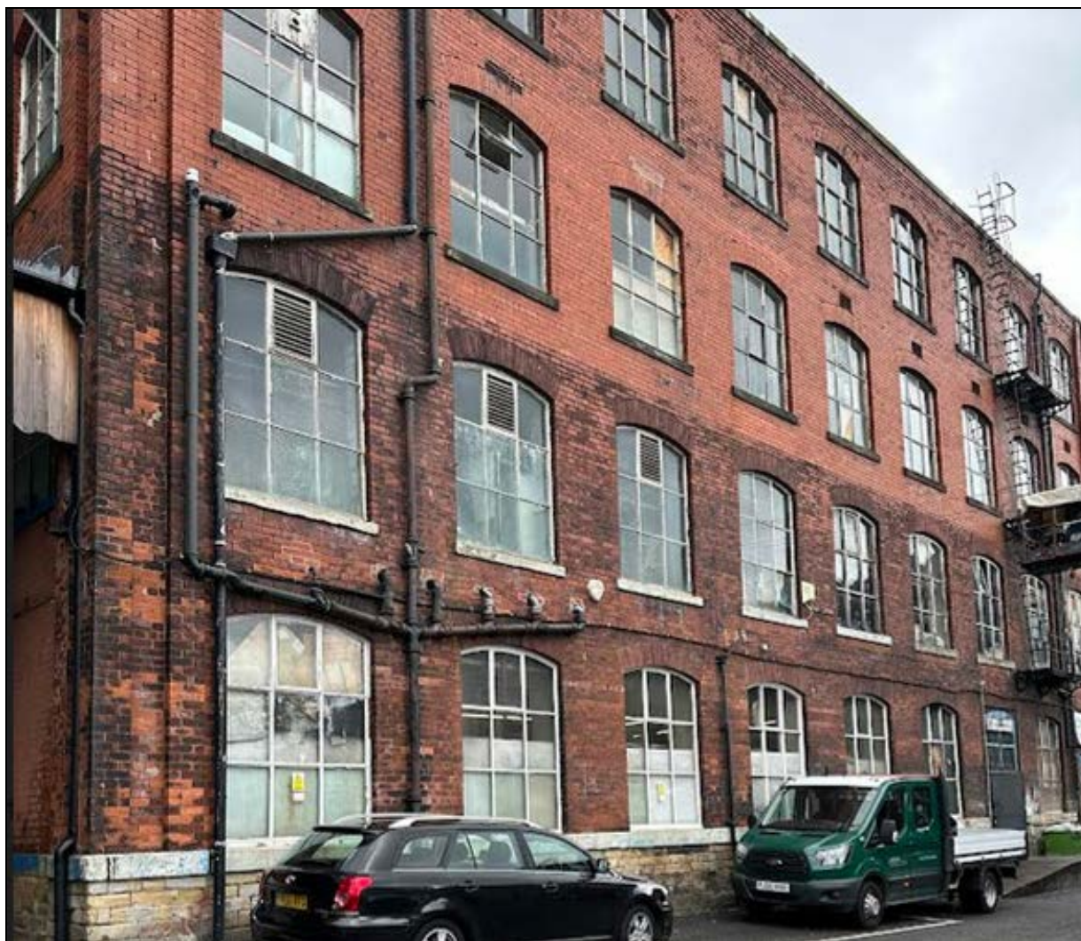
2. Southeast elevation of the mill, with units 30 (first six bays) and 31 (remaining three bays) on the ground floor
