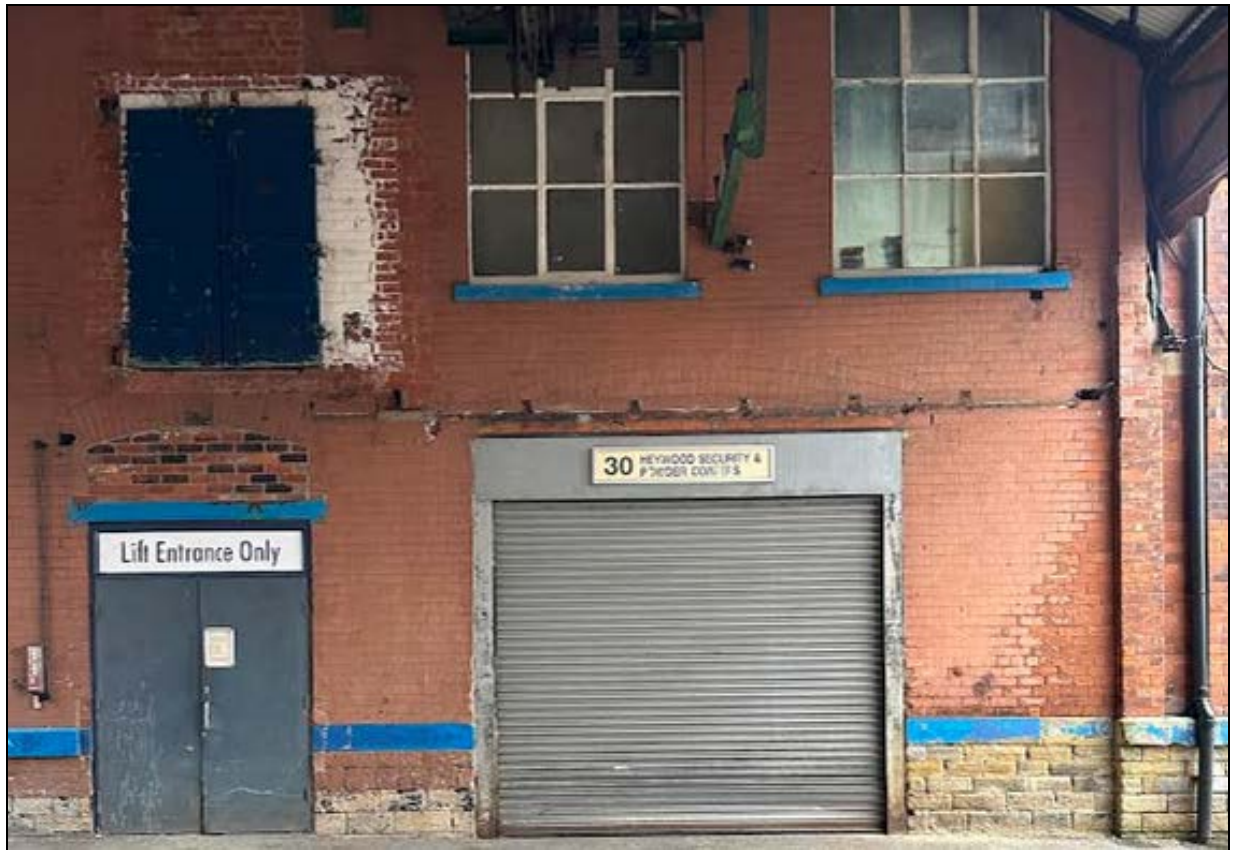
3. Roller-shutter doorway in southwest end of Unit 30
