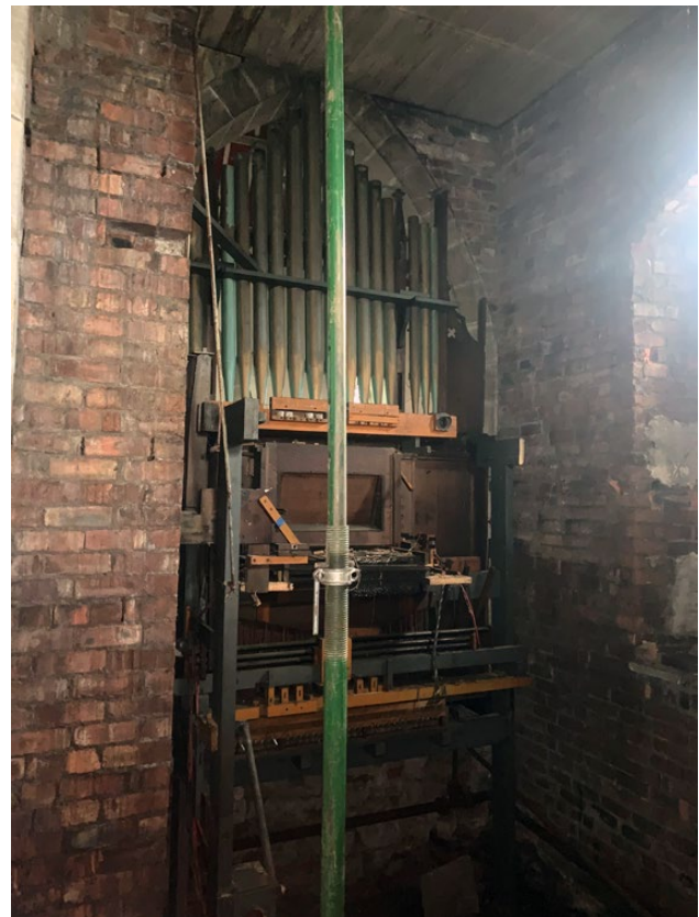
Remaining part of the Organ in Organ Chamber.
