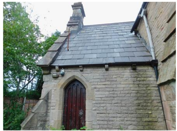
PHOTO 22 North-eastern Corner of Office
