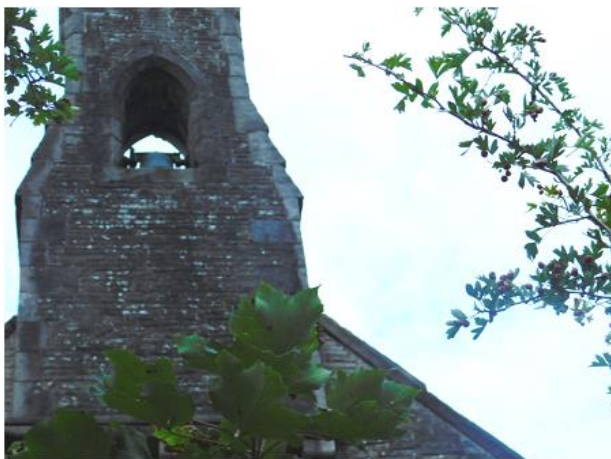
PHOTO 1 Western View of Bell Tower
