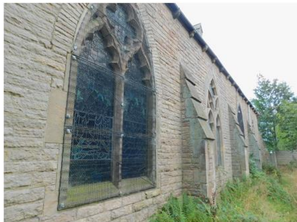
PHOTO 29 North-eastern View Along Nave
