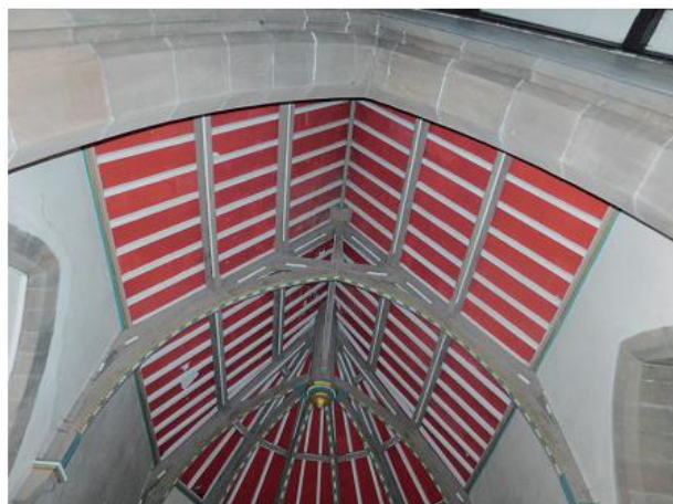
PHOTO 35 Underside of Tower Roof
