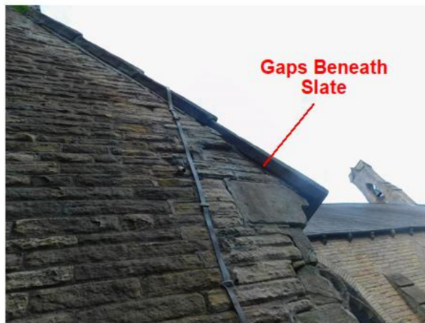
PHOTO 27 Junction of Vestry and Nave
