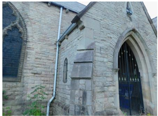
PHOTO 8 Southern Elevation of Entrance Porch
