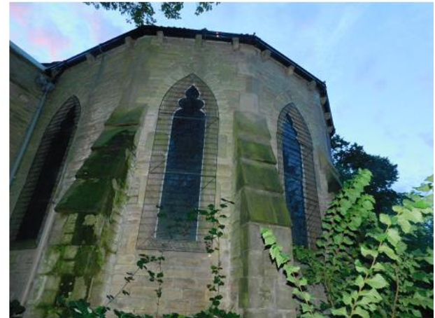
PHOTO 18 Southern Elevation of Tower
