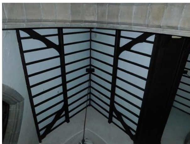
PHOTO 34 Underside of Transept Roof
