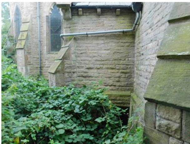
PHOTO 21 North-eastern Corner of Tower
