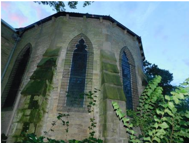
PHOTO 19 South-eastern Corner of Tower
