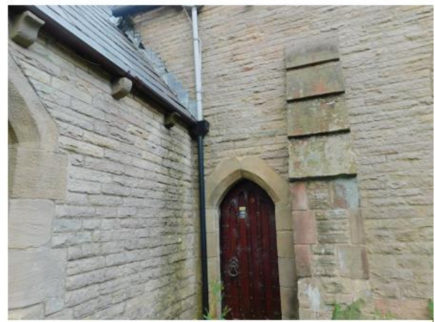
PHOTO 28 Western Elevation of Vestry
