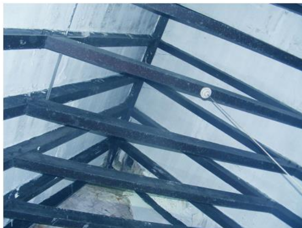
PHOTO 36 Underside of Chapel Roof
