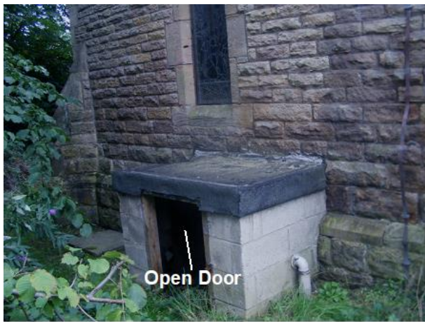
PHOTO 25 View of Storage Shed
