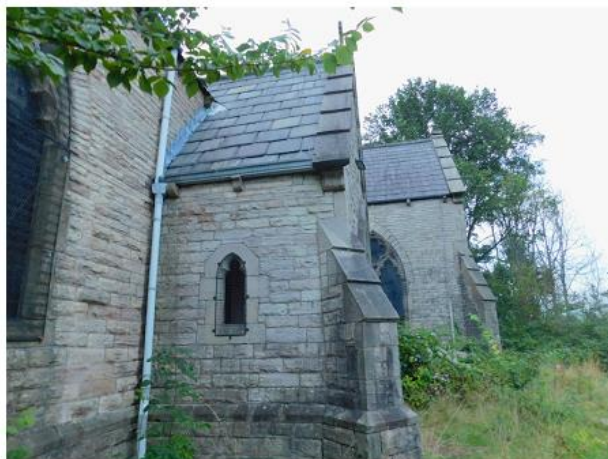
PHOTO 6 Western Elevation of Entrance Porch
