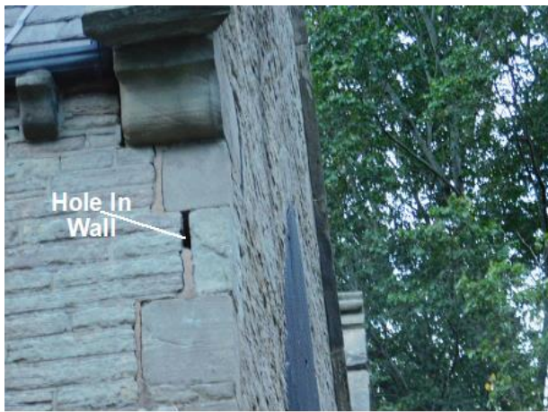
PHOTO 7 South-western Corner of Entrance Porch
