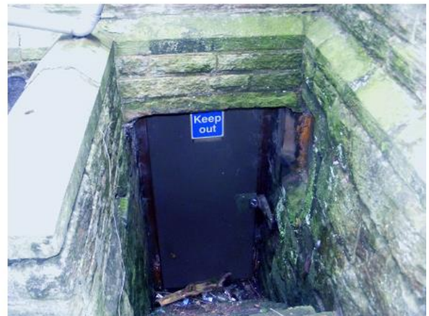
PHOTO 24 View of Locked Cellar Door
