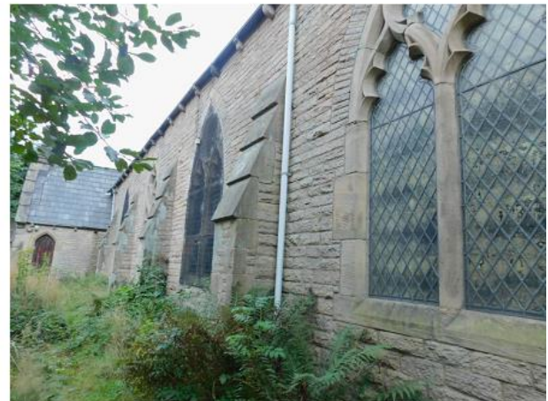
PHOTO 30 North-western View Along Nave
