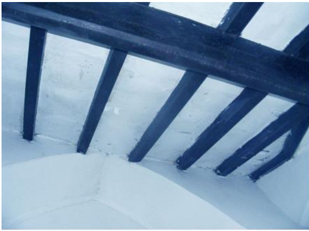
PHOTO 37 Underside of Office Roof
