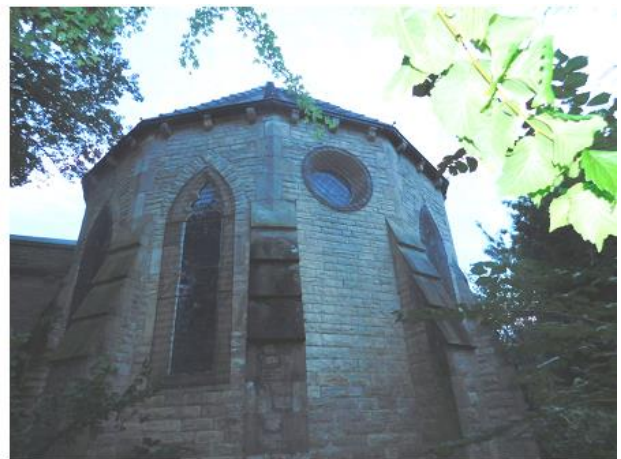
PHOTO 20 Eastern Elevation of Tower
