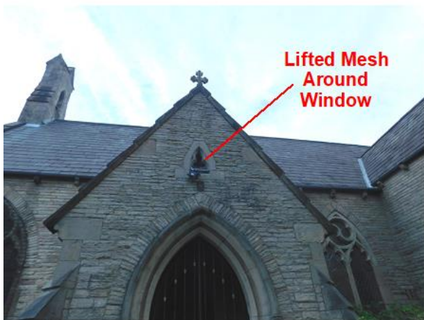
PHOTO 9 View of Southern Gable Over Entrance
