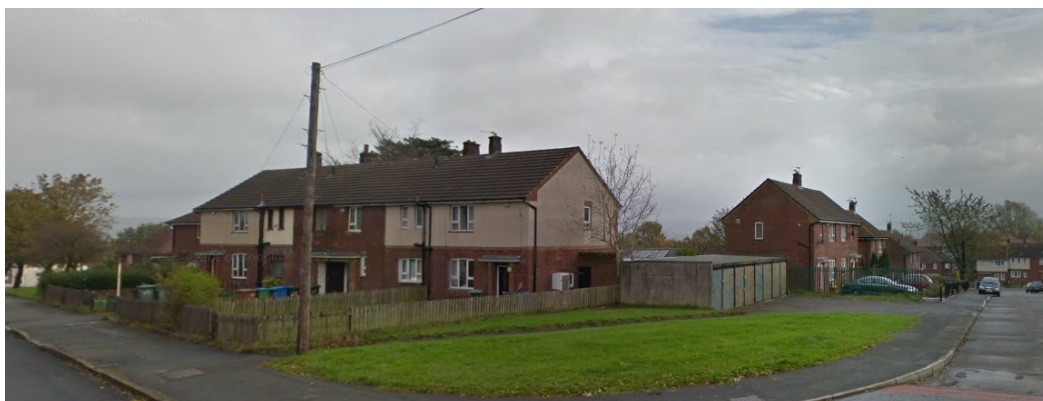
Image 2: Garage court on the corner of Hill Top Drive and Romney Avenue.
