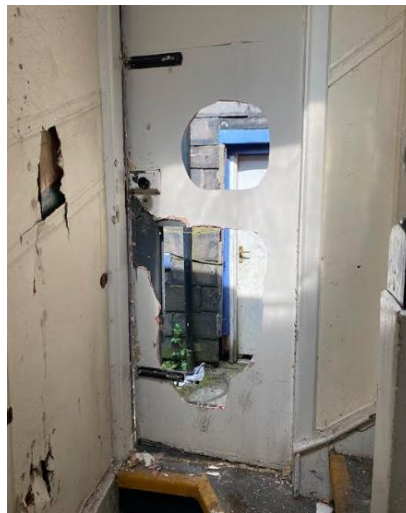
Pl.6: Altered stair and inserted partitions on the ground floor.
