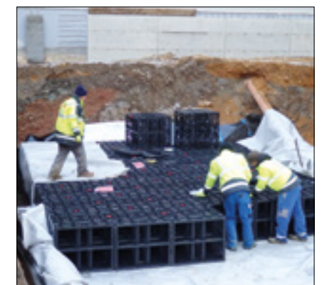
Industrial building, Tumeltsham (AT)
