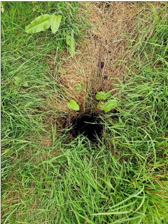
MH3 Location View
