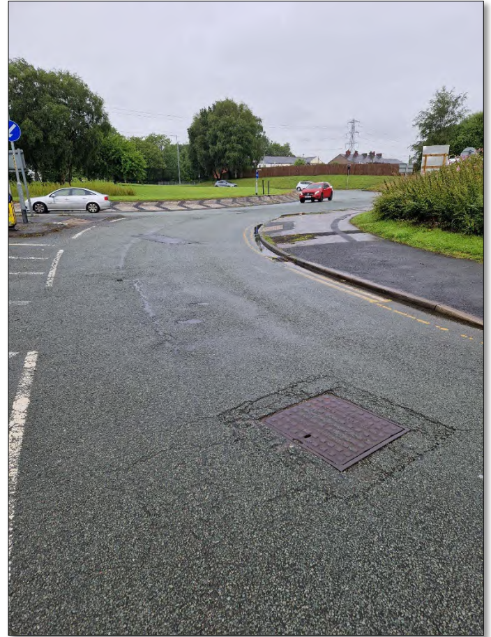
Manhole S8 Location View
