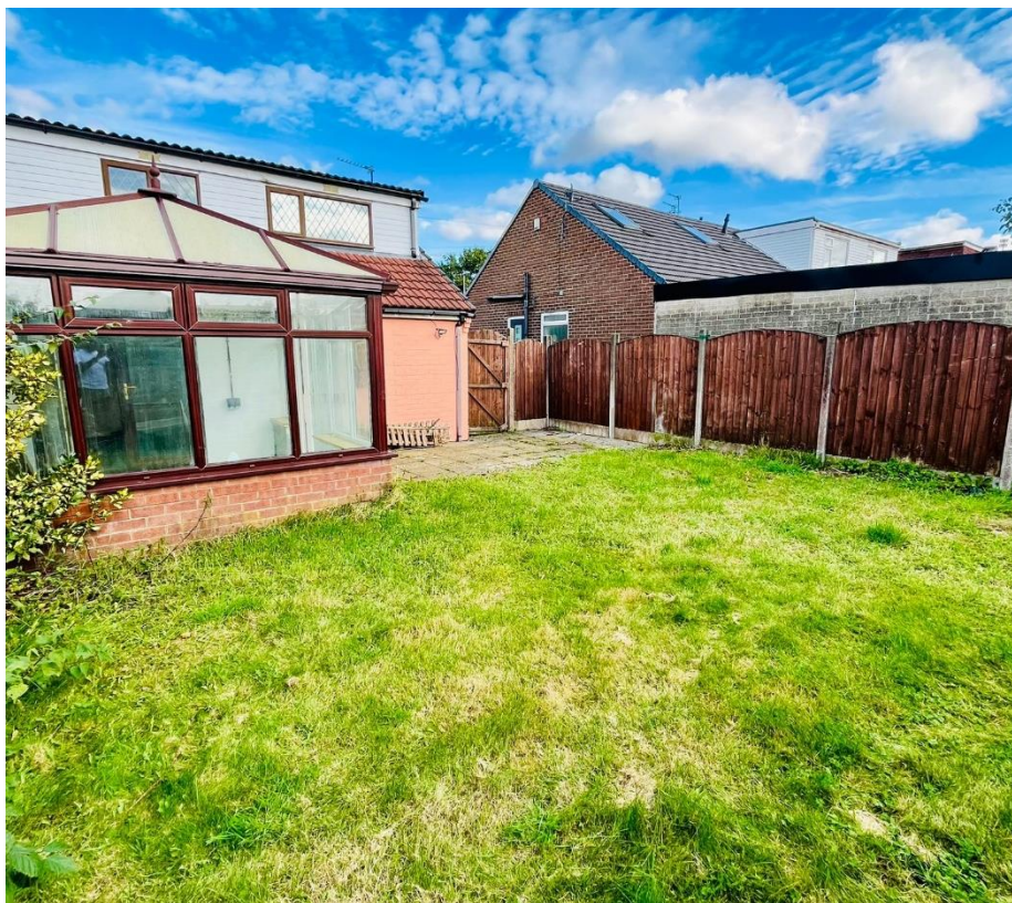
Photo 3: showing rear garden and back gate
