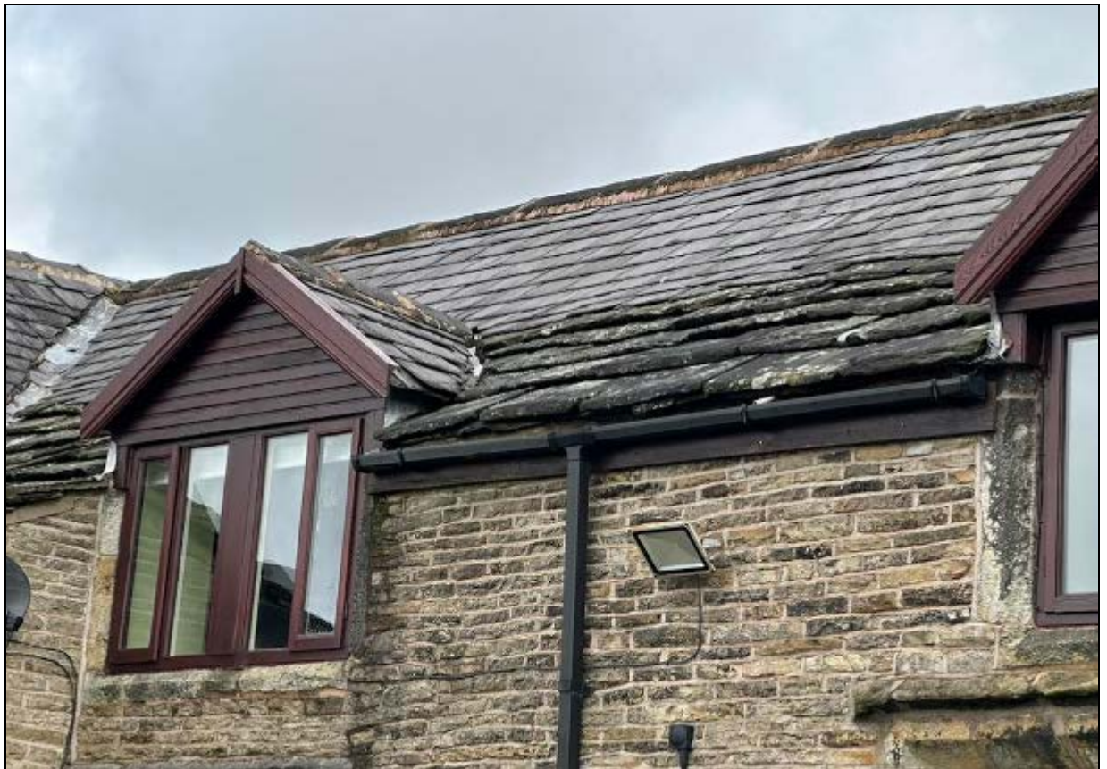
4. The roof is now mostly slate with areas of stone flag remaining at the front
