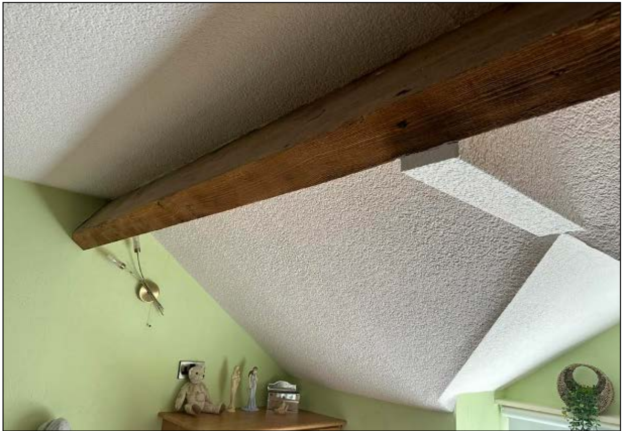
6. Visible roof beams are not original
