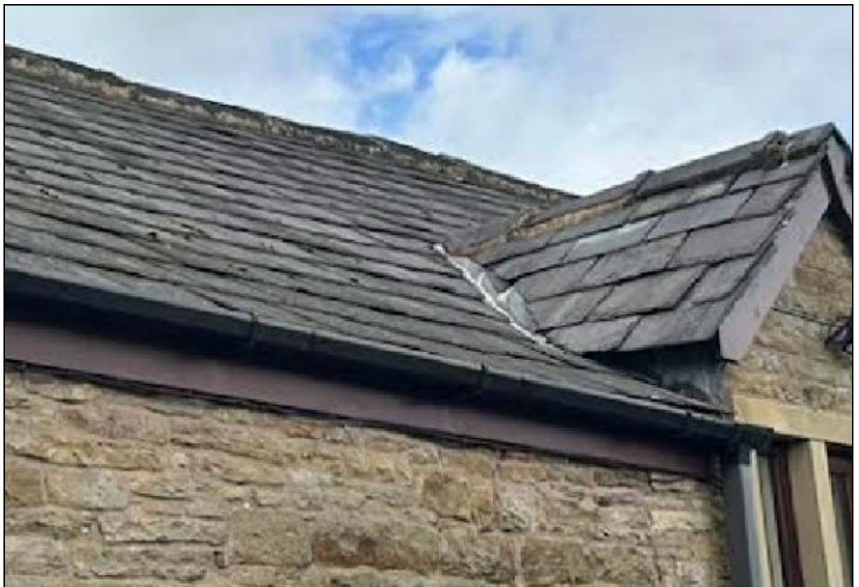
5. Rear roof plane is covered with slate; change may have occurred when the dormers added
