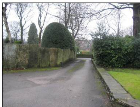
Figure 10: Stone boundary walls forming the west boundary to the front of the site.
