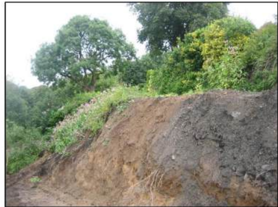
Figure 31: Planting and vegetation between the proposed development site and Hill House.
