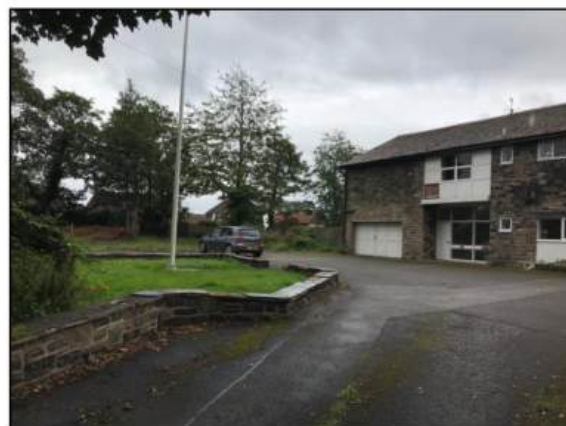
Figure 8: View of the location of the demolished stables building showing the relationship with Stable Hills.
