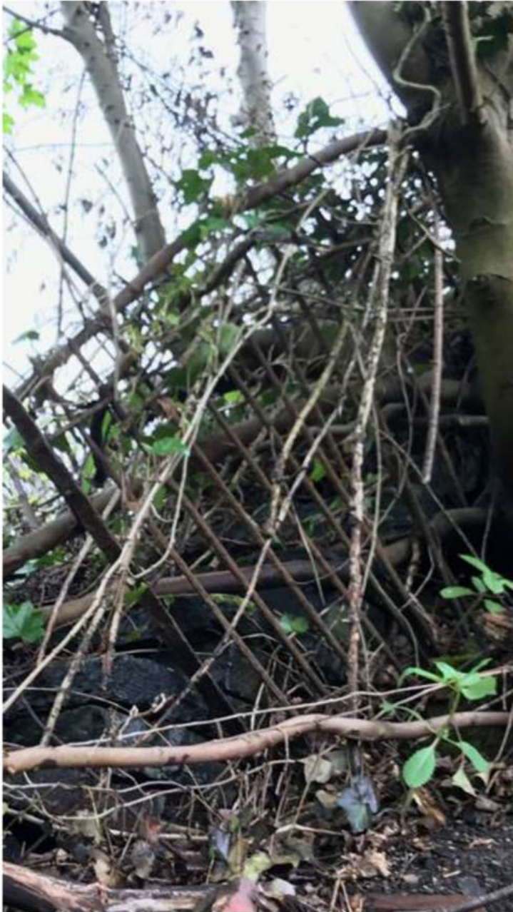
Cast iron guard rail
