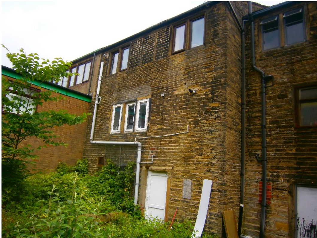
Rear elevation of no. 108 Dale Street: Hairdressers ground floor storage, Hairdressers first floor, living accommodation second floor
