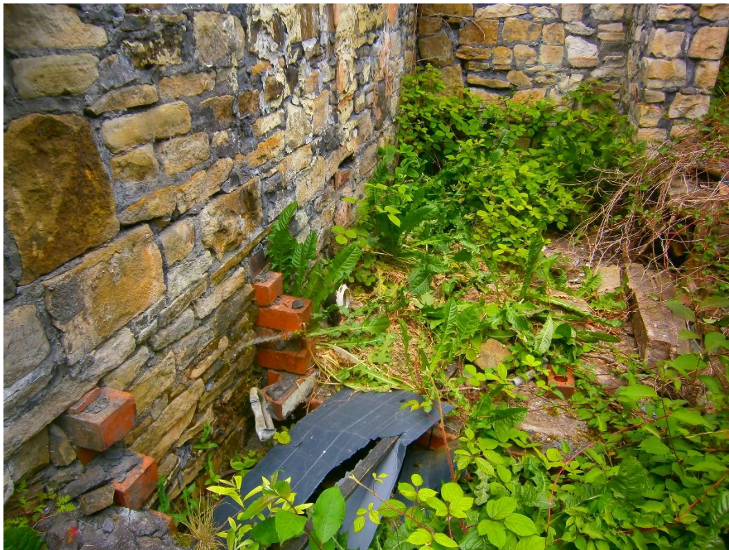
Drainage and water connection in demolished section of garage
