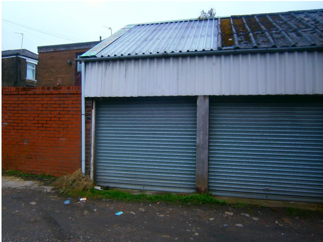
Existing garage front unit 1-2
