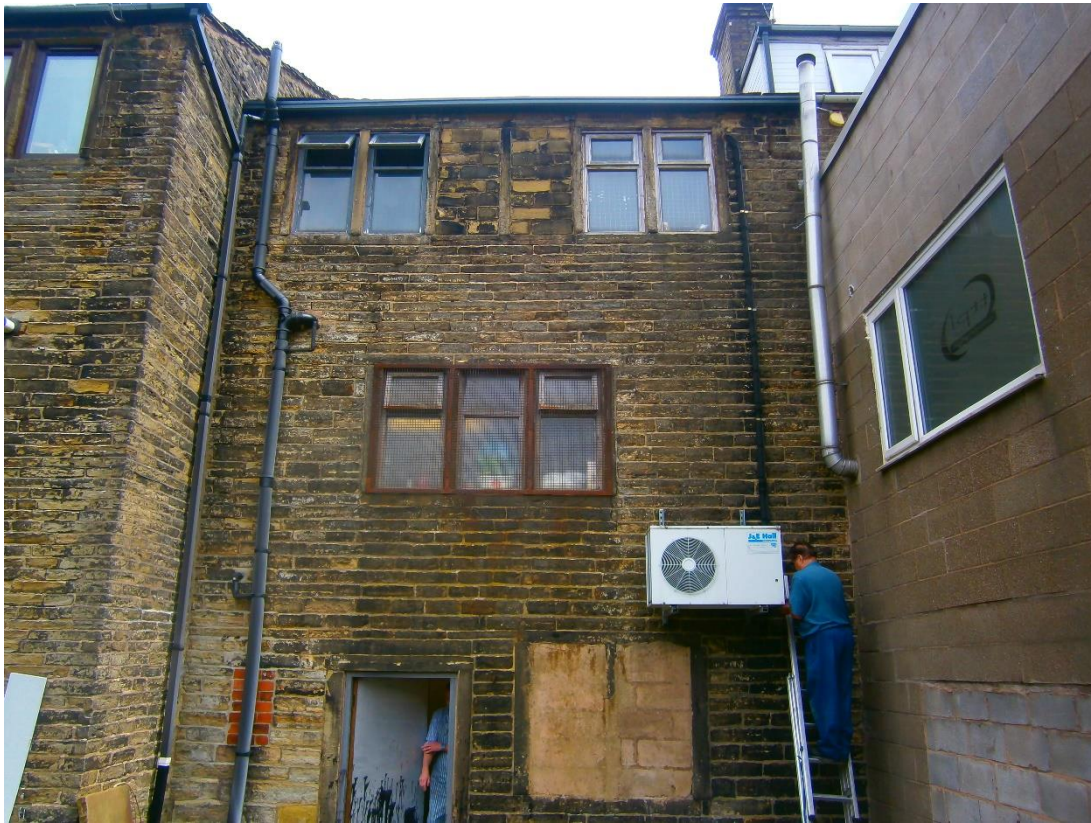
Rear elevation of no. 110 Dale Street: Butchers ground floor windows, Butchers cold room at first floor, Storage at second floor
