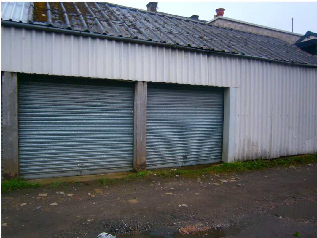
Existing garage front unit 2-3
