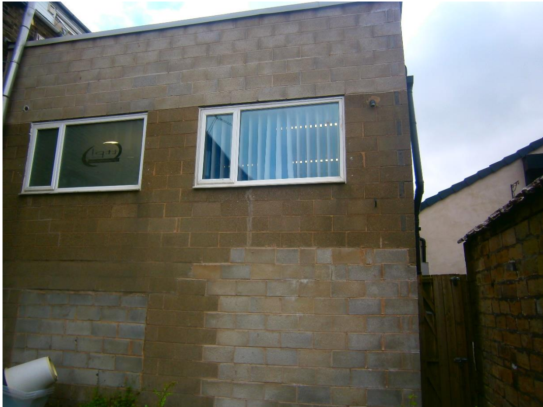
Side elevation of no. 112 Dale Street: Office windows at first floor
