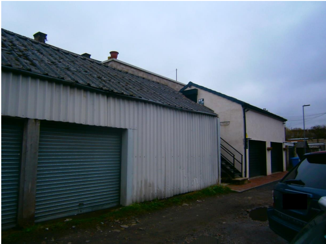
Existing garage front unit 3
