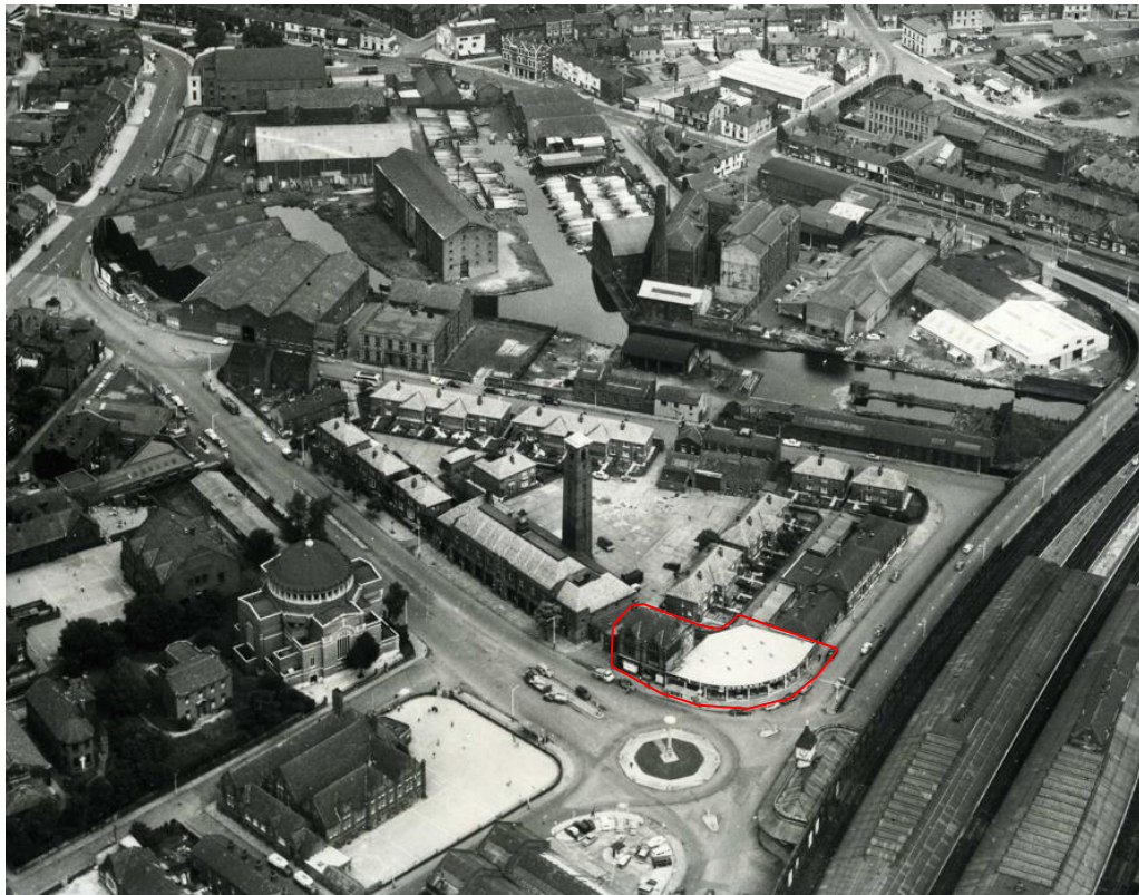
Figure 3.12: 1964 Aerial Photograph of Maclure Road (courtesy of Rochdale Local Studies). The location of the Site is outlined in red.
