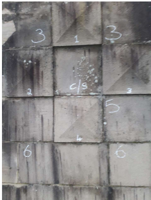
Referencing of the stonework prior to dismantling
