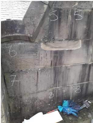
Referencing of the stonework prior to dismantling
