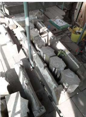
Stonework referenced and stored on the scaffolding-and at ground level and protected.
