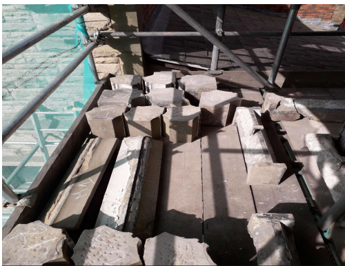
Stonework referenced and stored on the scaffolding-and at ground level and protected.
