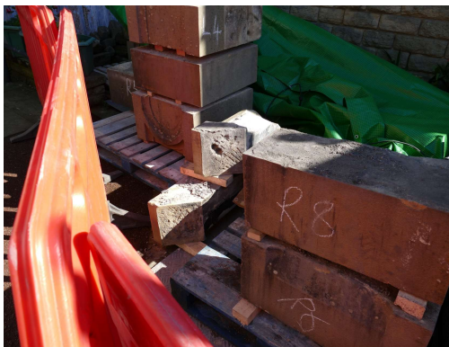
Stonework referenced and stored on the scaffolding-and at ground level and protected.
