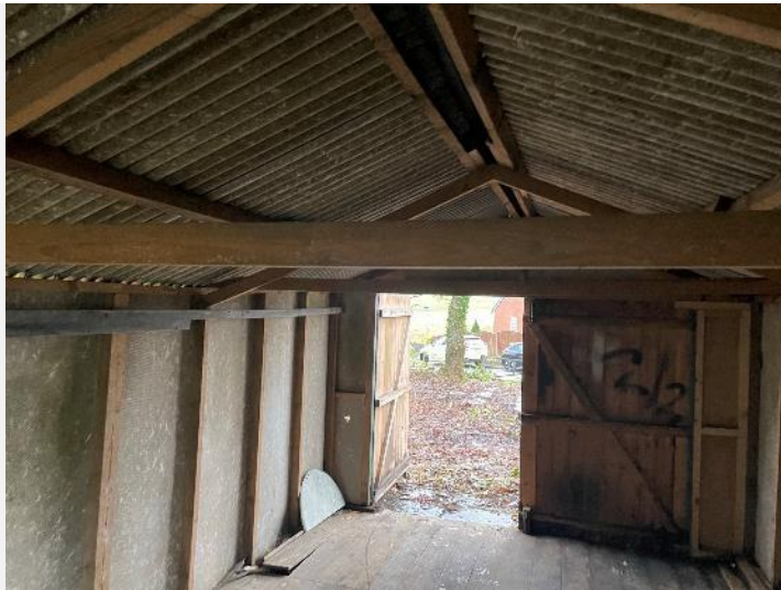
Photo 4. Internal view of Shed 3
