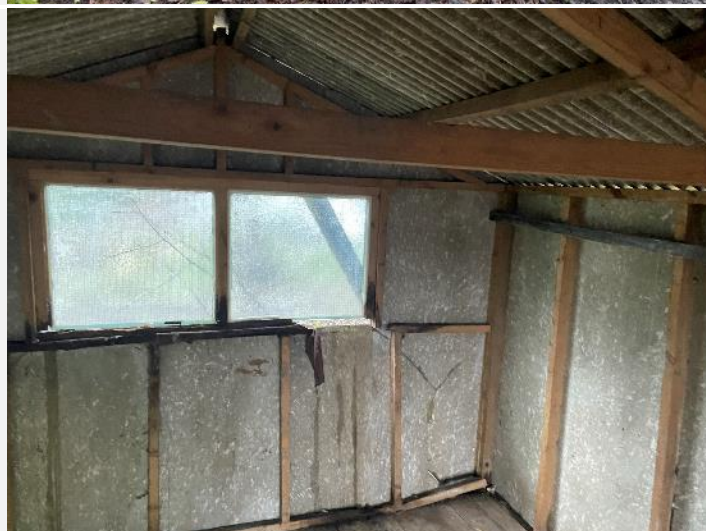
Photo 3. Internal view of Shed 3
